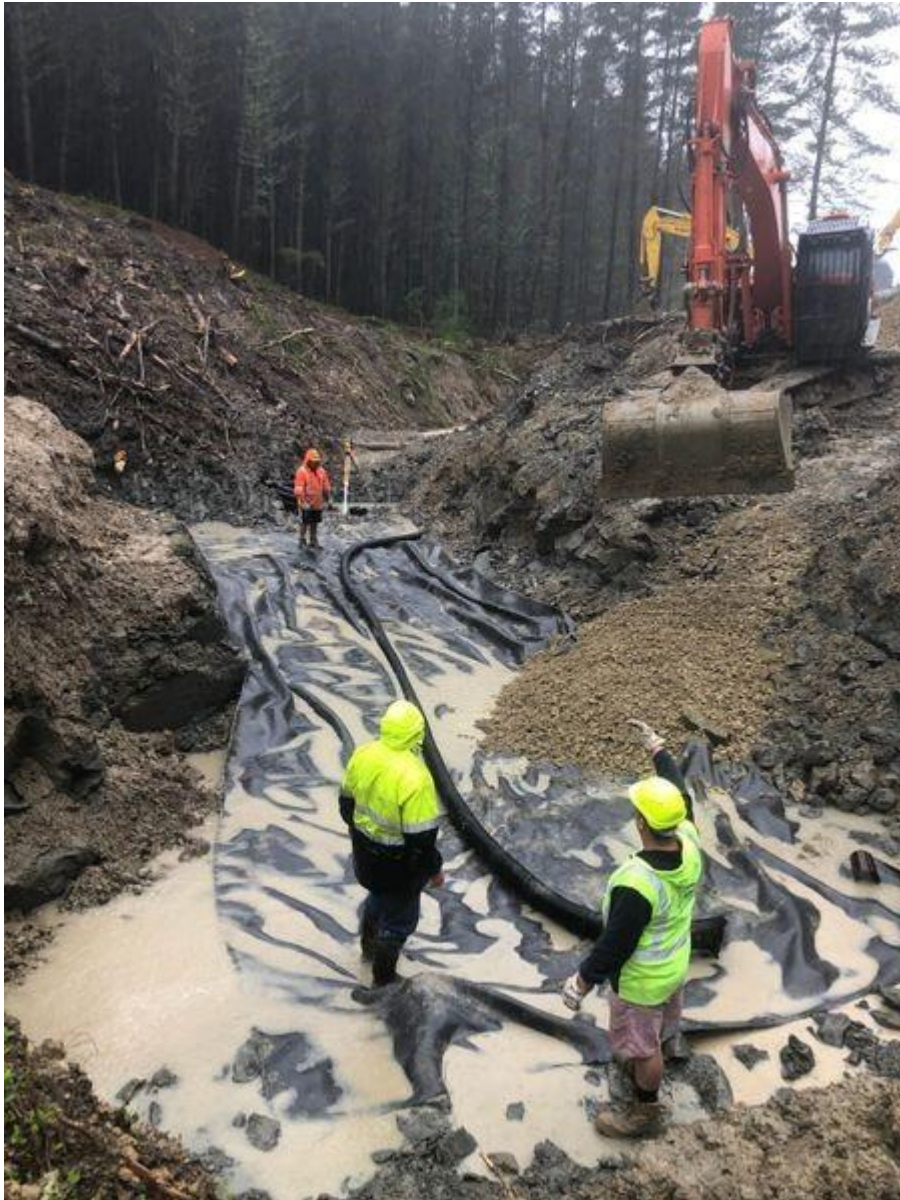
Photo 1: Installation of 2550 mm culvert.
