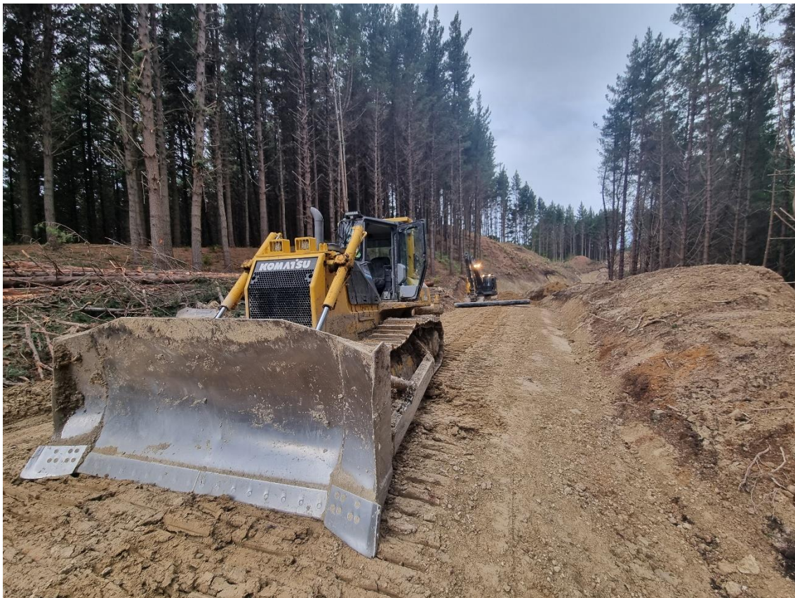
Photo 2: Roothing machinery finishing formation on Kiwi Road between Landings 41 and 45.
