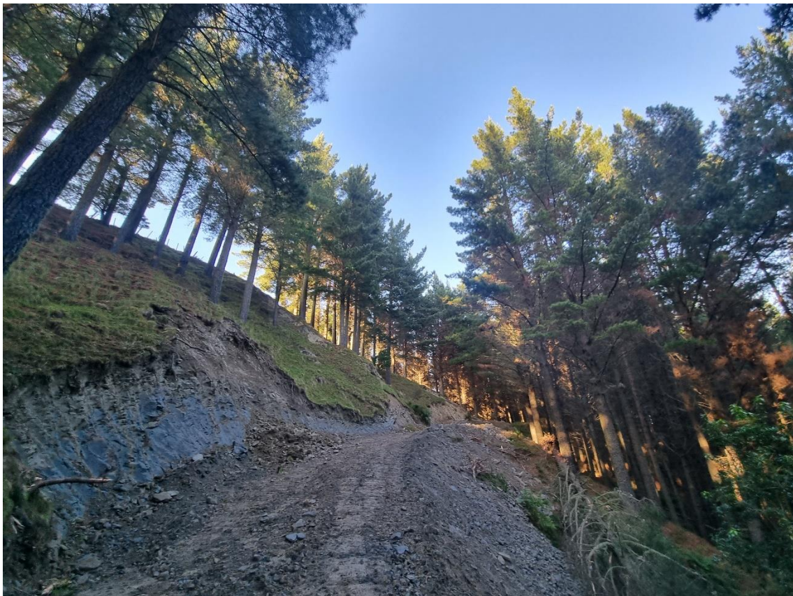
Photo 4: Skidder track put in ready for roadline operation extraction.
