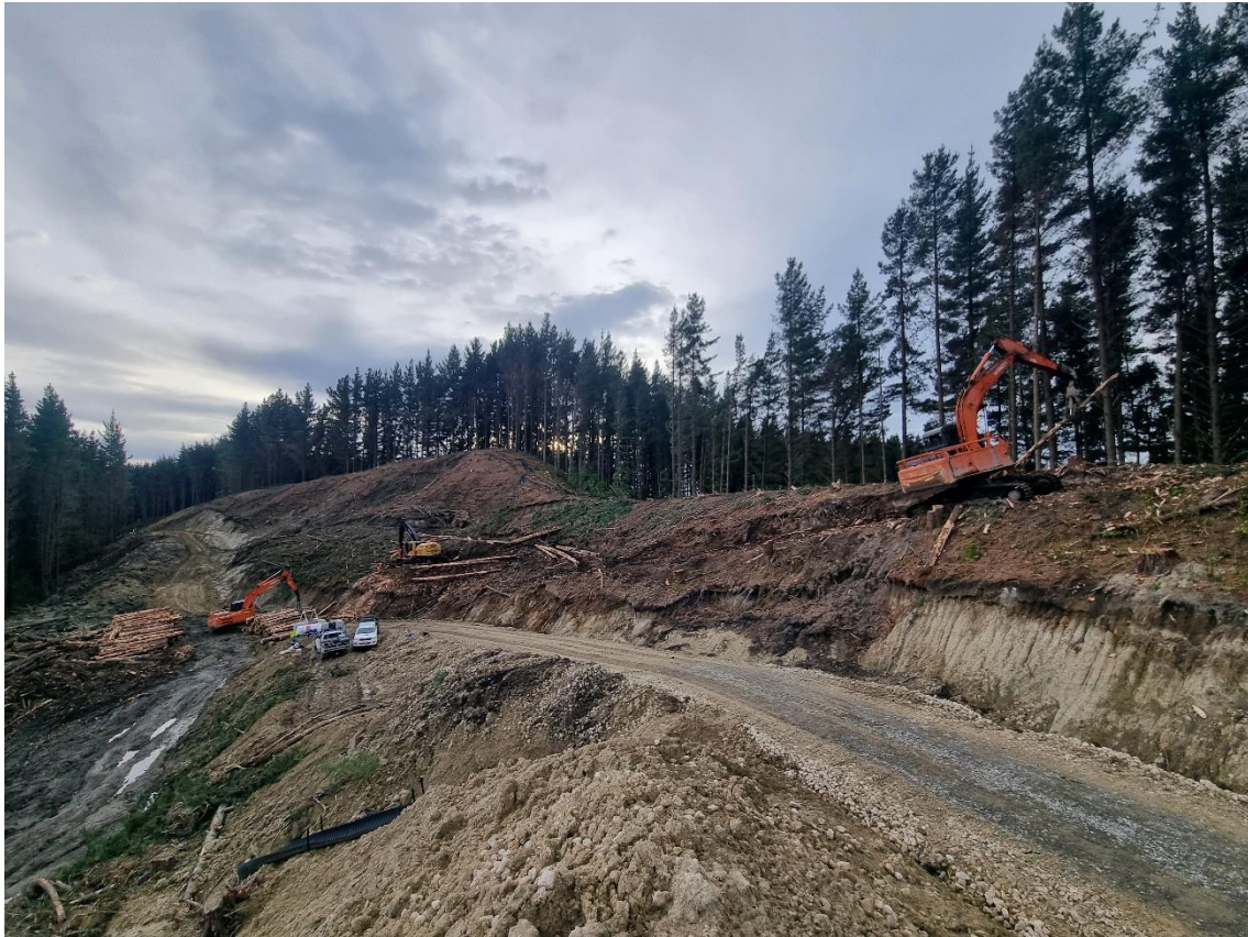
Photo 3: Crew removing small strip above protected native area.
