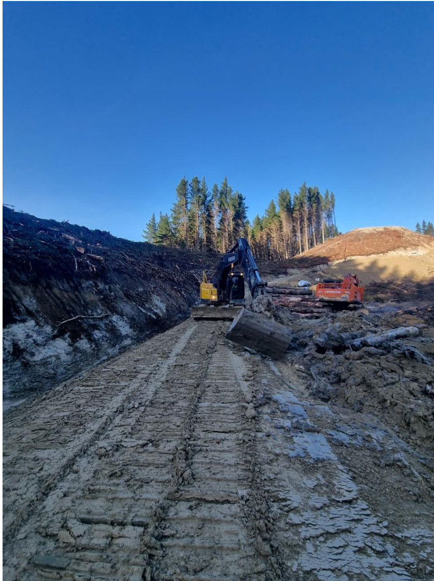
Photo 5: Earthworks widening section of road where Landing 41 was.
