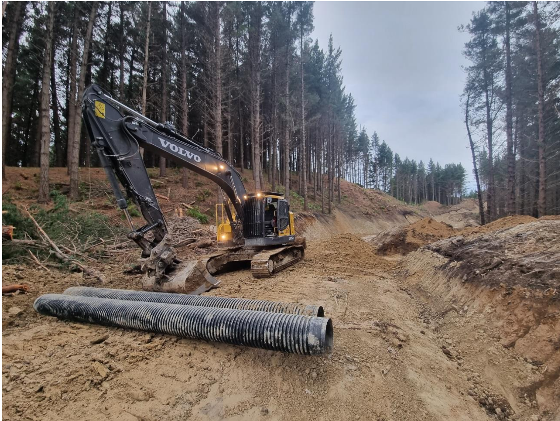
Photo 1: Digger installing cross road culverts on Kiwi Road.
