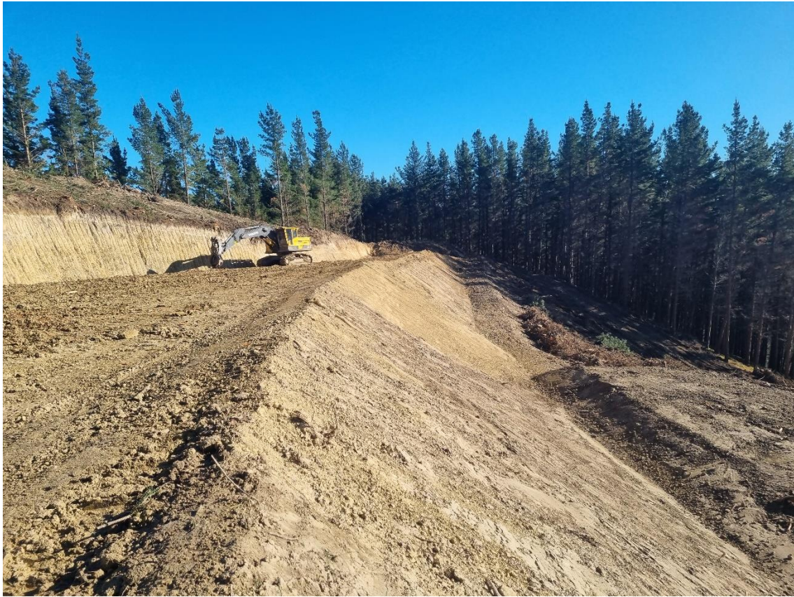
Photo 7: Landing 2 recently constructed by Tahurua Earthmovers.
