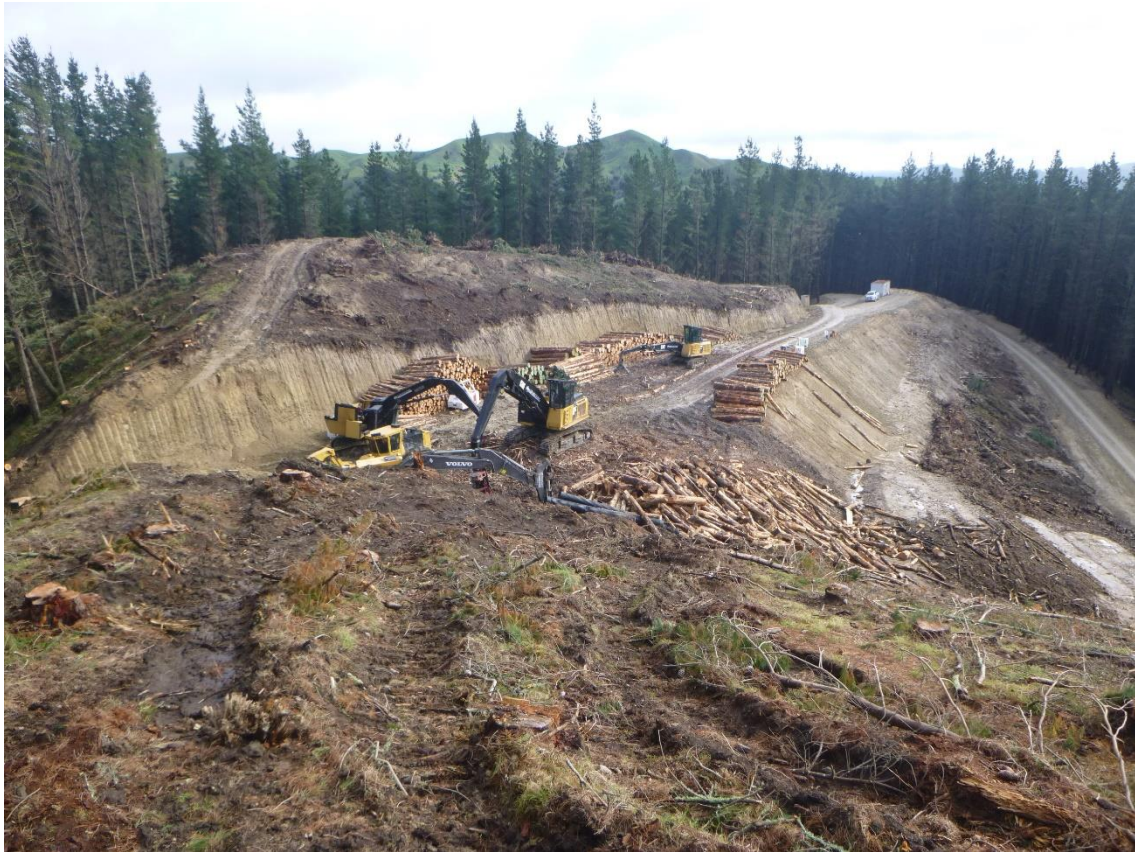
Photo 1: A & R Logging crew, Log 19 operating on Landing 2 - processing logs.
