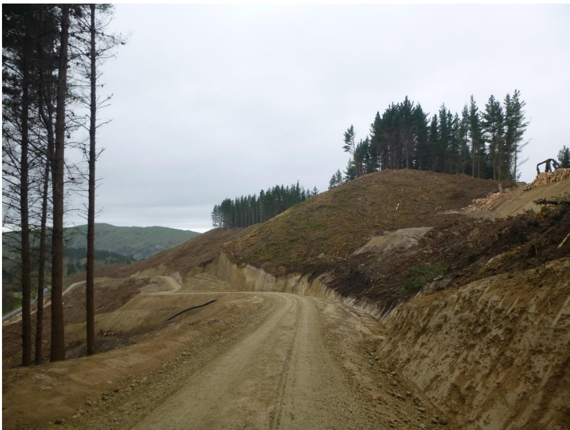
Photo 12: Tahurua Earthmovers - formed and metalled section of Mad Mutt Road above the 1km marker.
