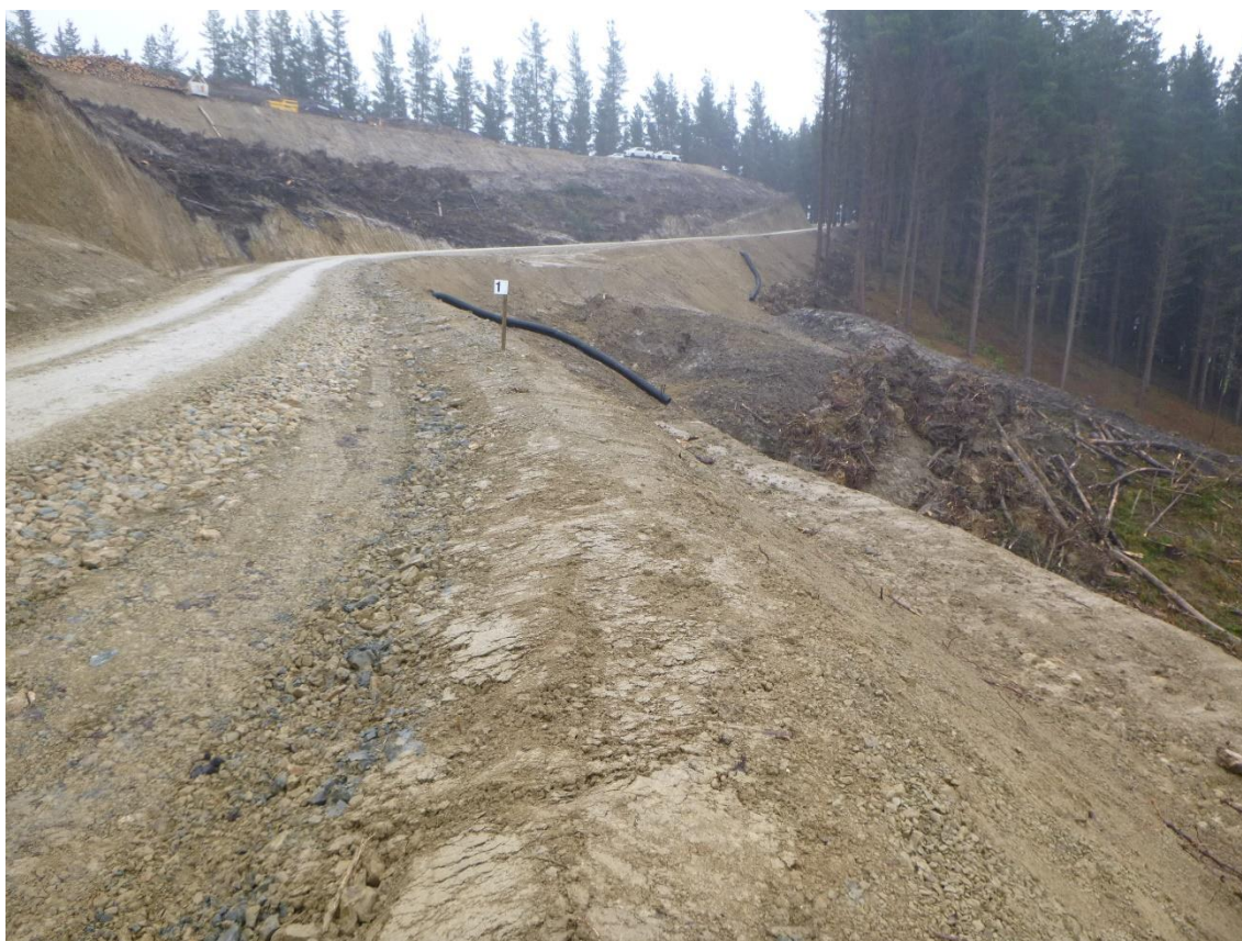
Photo 10: Tahurua Earthmovers - formed and metalled section of Mad Mutt Road at the 1km marker.
