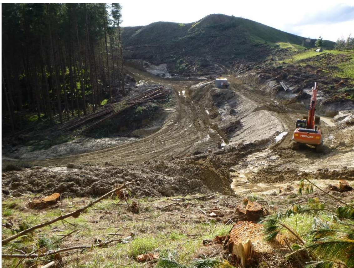
Photo 9: Tahurua Earthmovers constructing the intersection of Mad Mutt Road and Wood Road.
