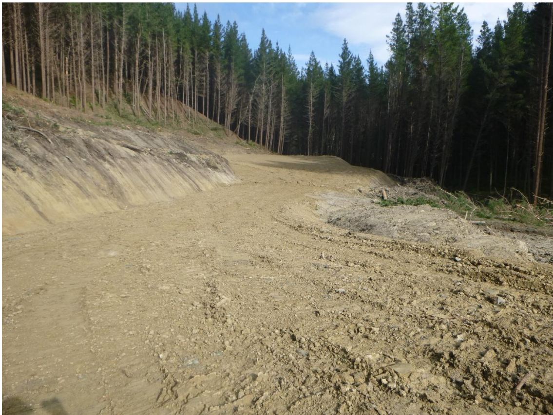
Photo 8: Landing 3 constructed by Tahurua Earthmovers.
