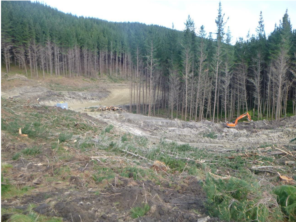
Photo 13: Tahurua Earthmovers – rehabilitating the pull track used by A & R Logging in Setting 500 near Landing 3.
