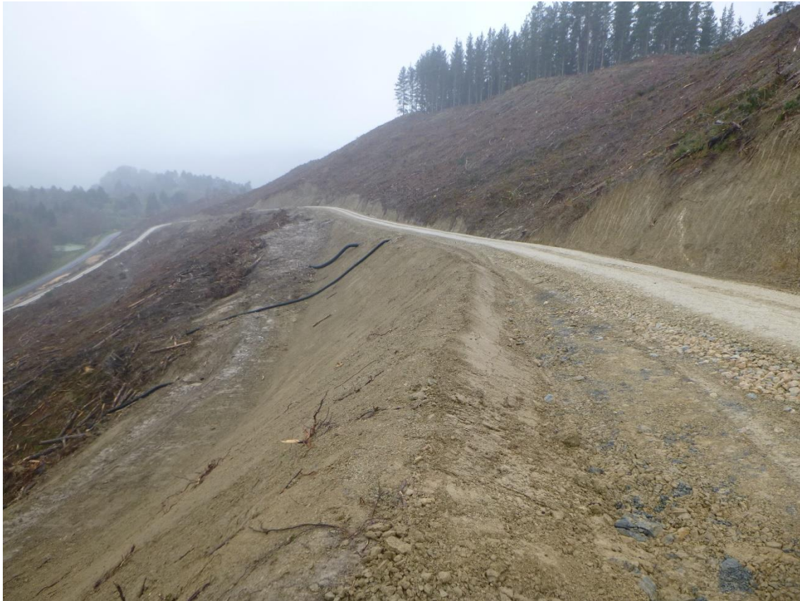
Photo 11: Tahurua Earthmovers - formed and metalled section of Mad Mutt Road below the 1km marker.
