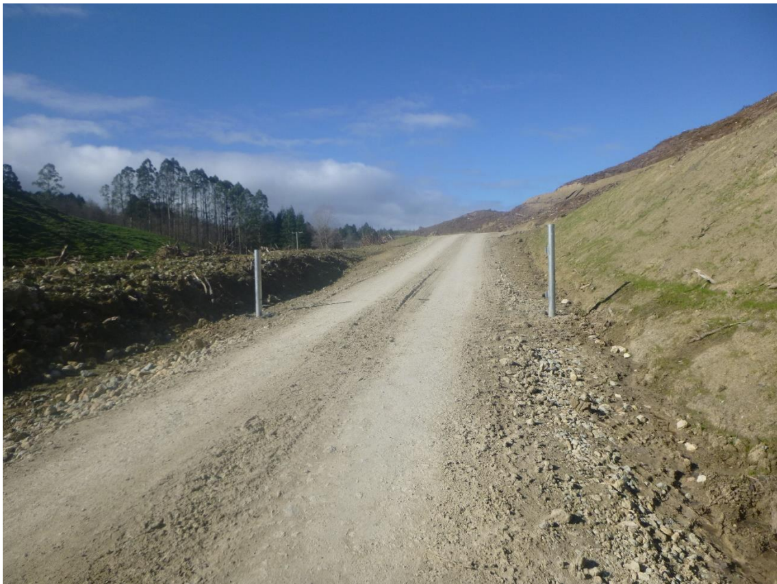
Photo 14: Posts for a security gate to be installed at the start of Mad Mutt Road.
