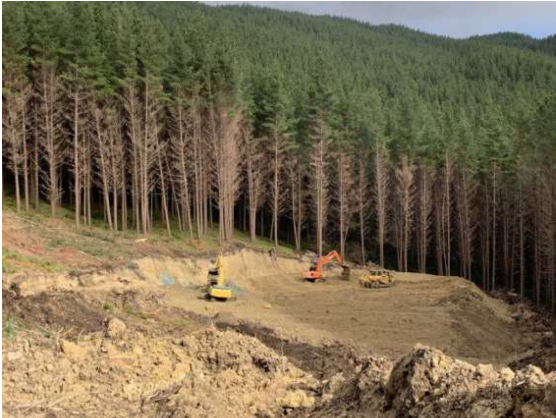
Photo 1: Tahurua Earthmovers building Landing 43 which is half in Portobello Forest and half in Monterey Forest.
