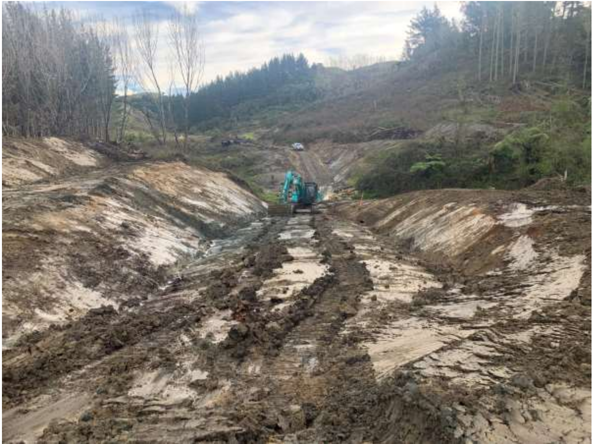
Photo 1: Construction of Griffiths Road over the river crossing.
