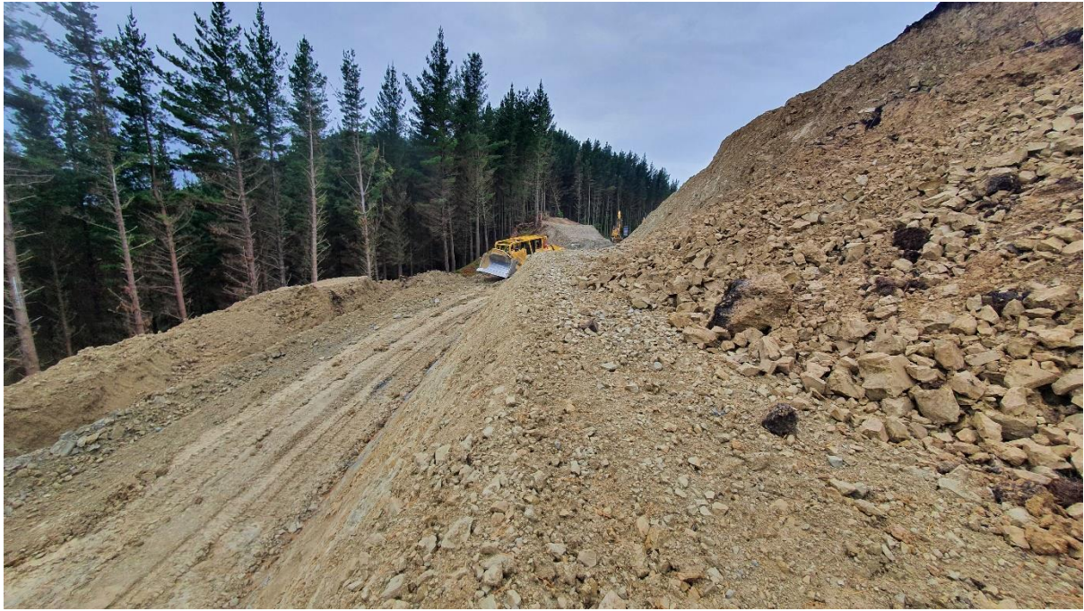
Photo 1: D8 machine undertaking final tie in works on Sylvan Road to Landing 13 on roadline Setting 504.
