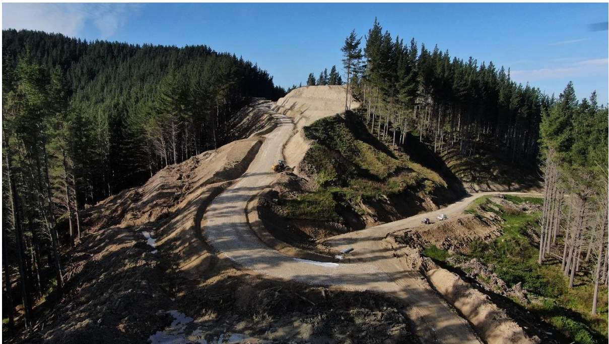
Photo 4: Pavement on Sylvan Road nearing completion.
