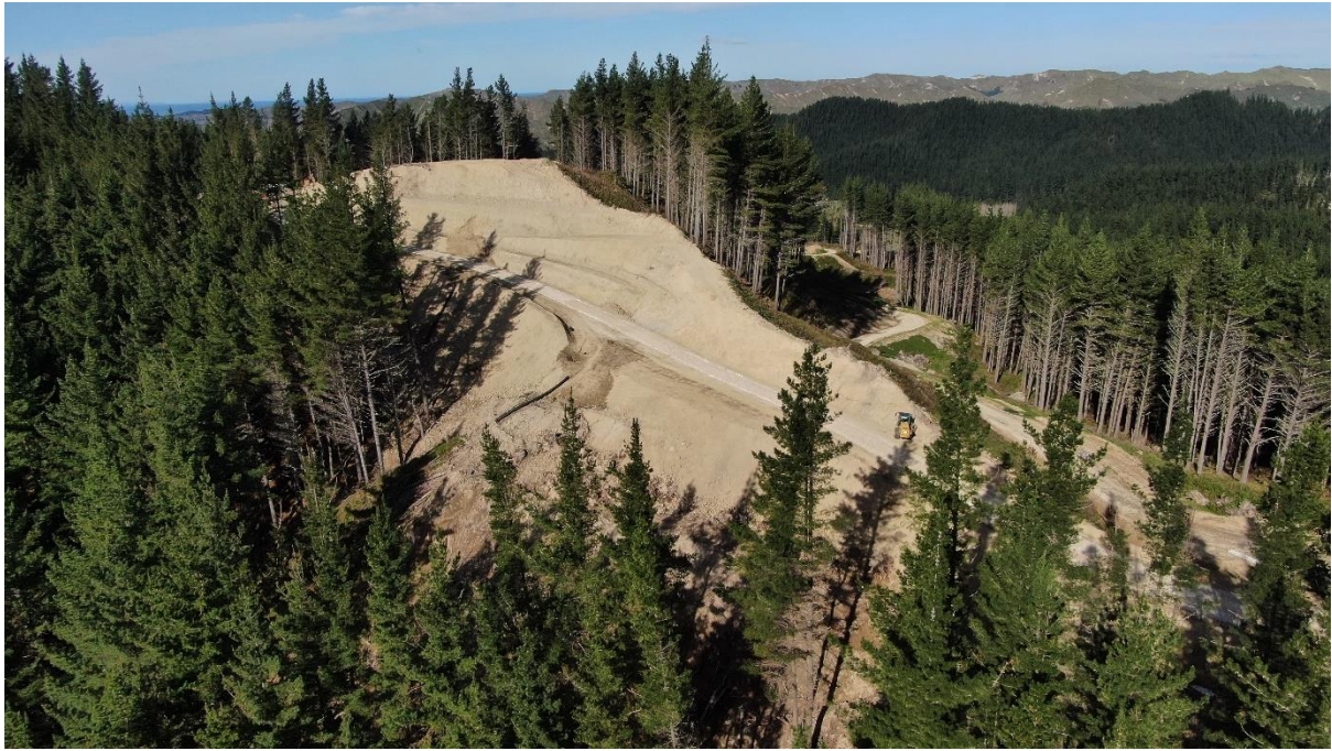
Photo 3: Pavement on Sylvan Road, roadline Setting 504 showing water controls and benching practices.
