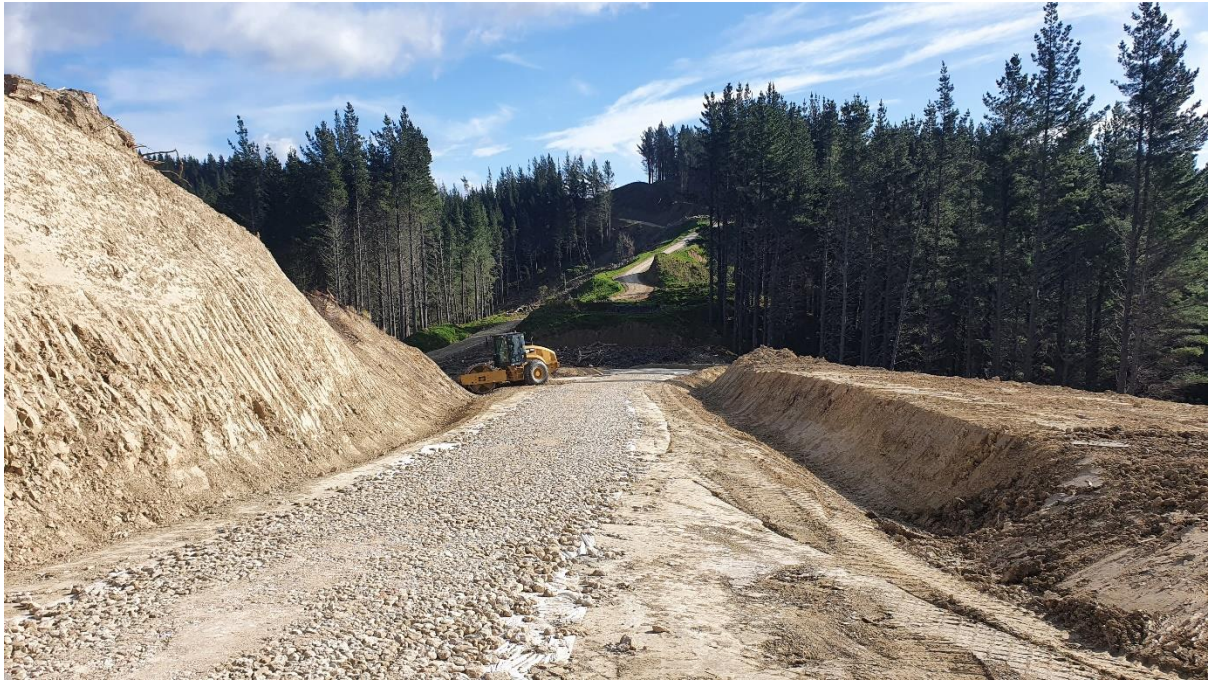
Photo 5: Placing sub-base and compacting on Sylvan Road.
