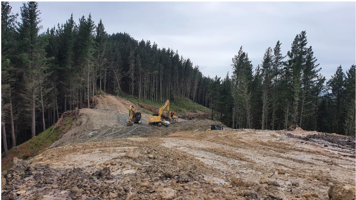
Photo 2: Earthworks crew undertaking final shaping works on Landing 13.
