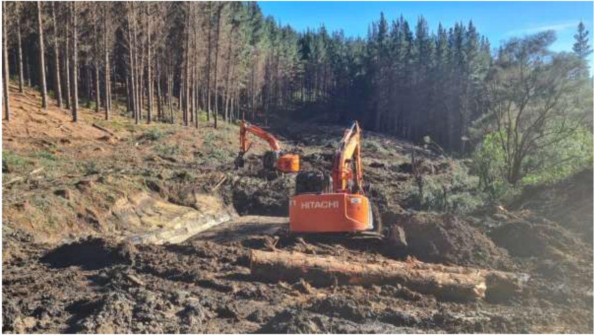
Photo 5: Landing 61 being formed.
