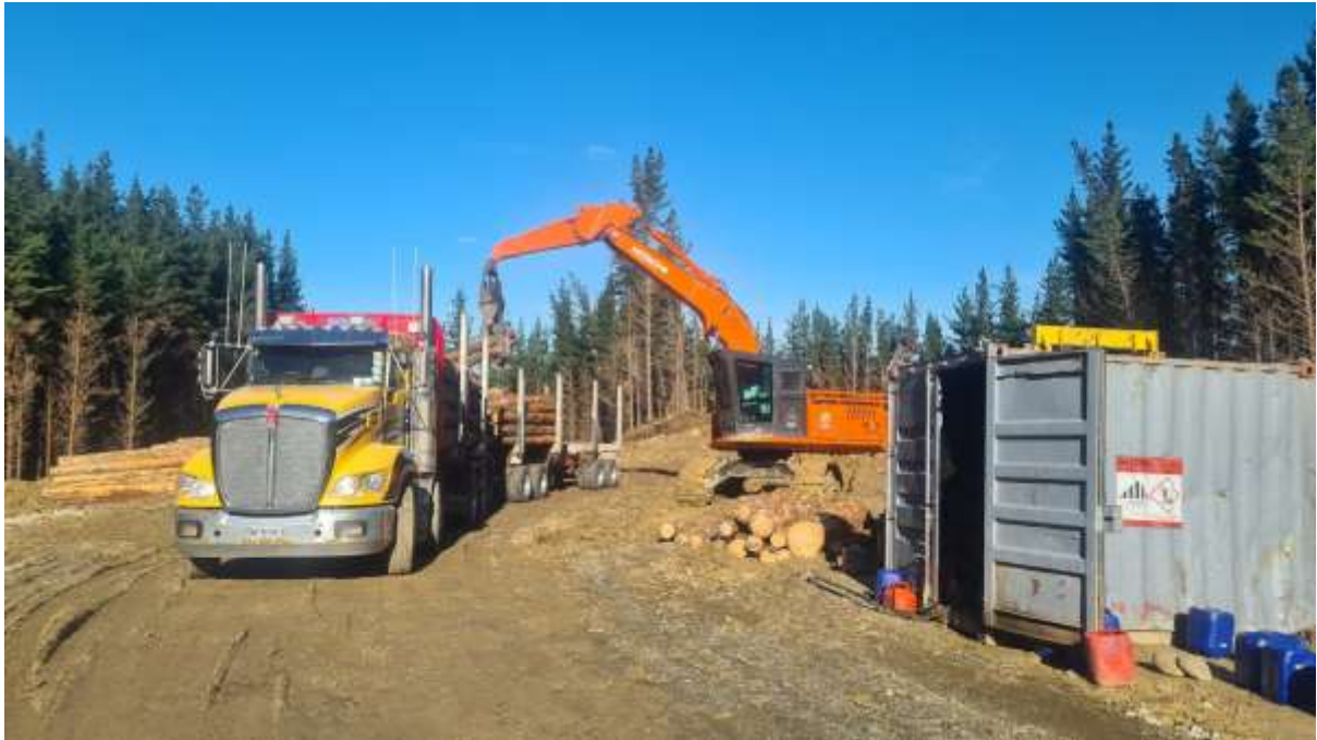
Photo 1: Loading up a truck on Landing 61.
