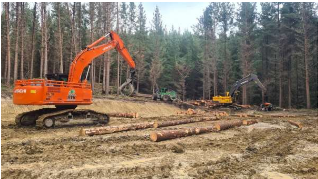
Photo 2: Loadout machine setting out the loadout bay on Landing 61.
