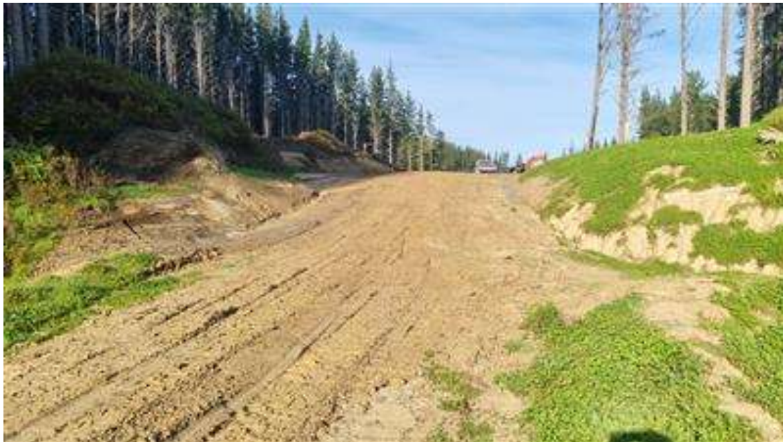
Photo 1: Yeoman Road maintenance - section of road between Landings 4 & 5 that has just been reshaped due to heavy rain event.
