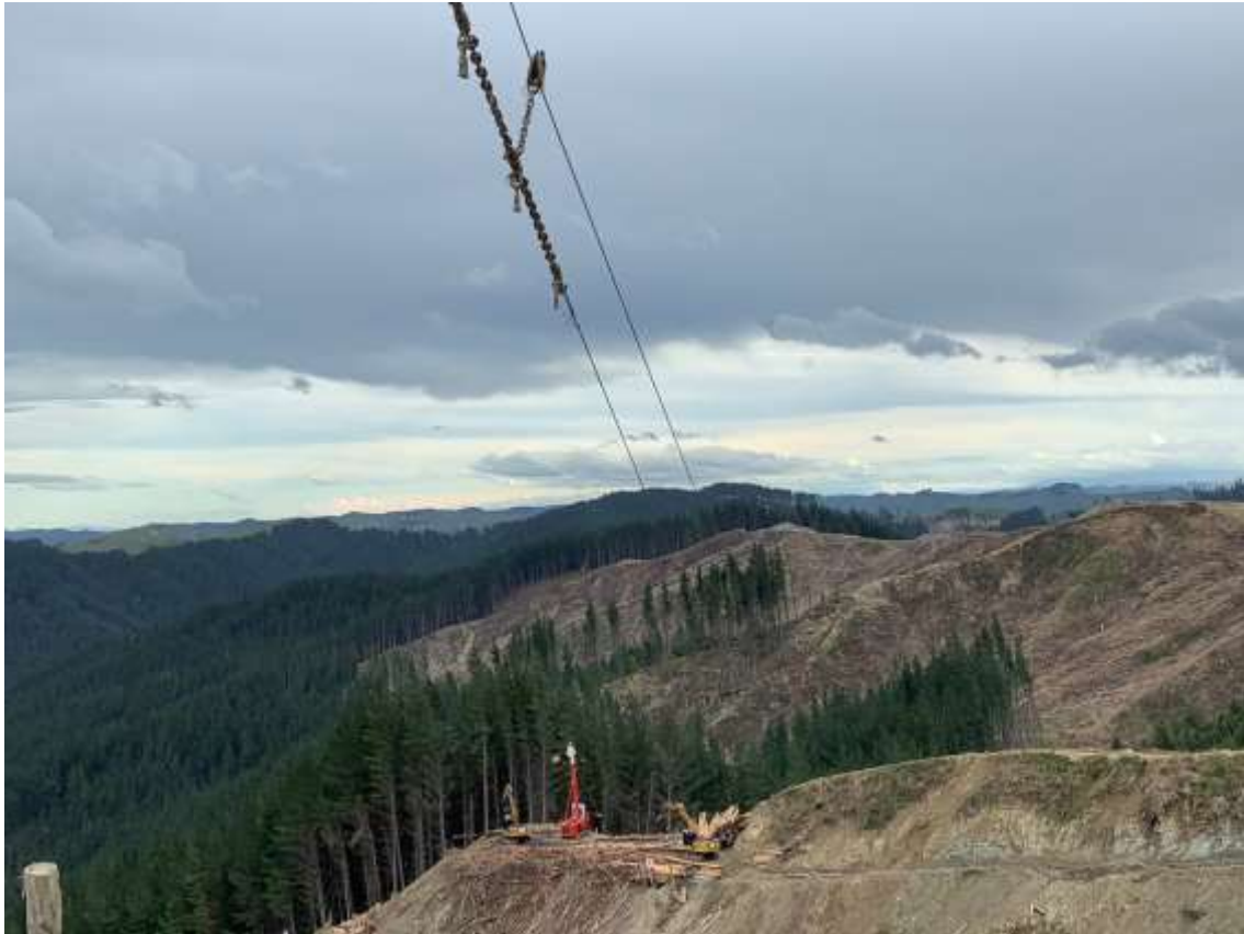
Photo 5: Madill 171 ropes set up for two-stage from Landing 605.
