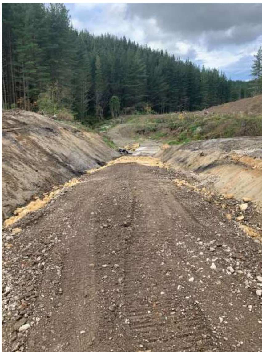
Photo 3: Griffiths Road, Setting 500 - river crossing approaches under construction.
