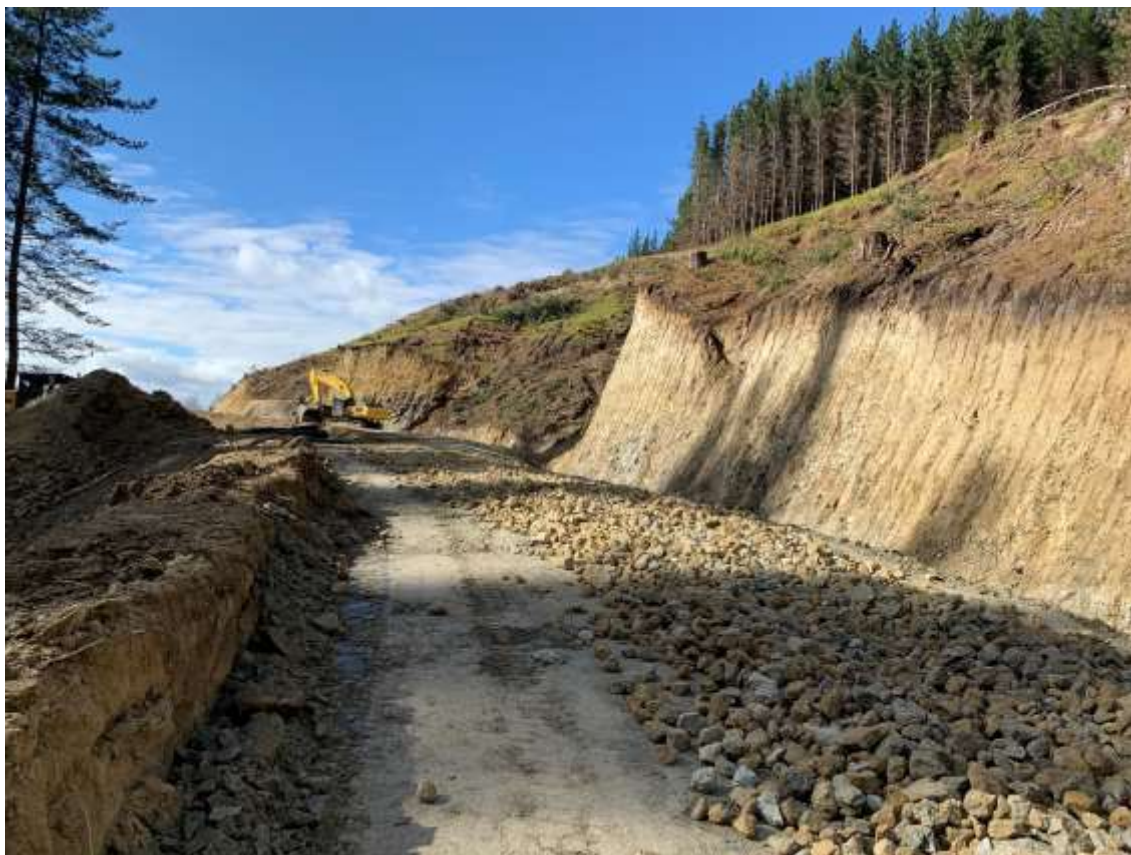
Photo 6: Clarke Road metalling to the crossing.
