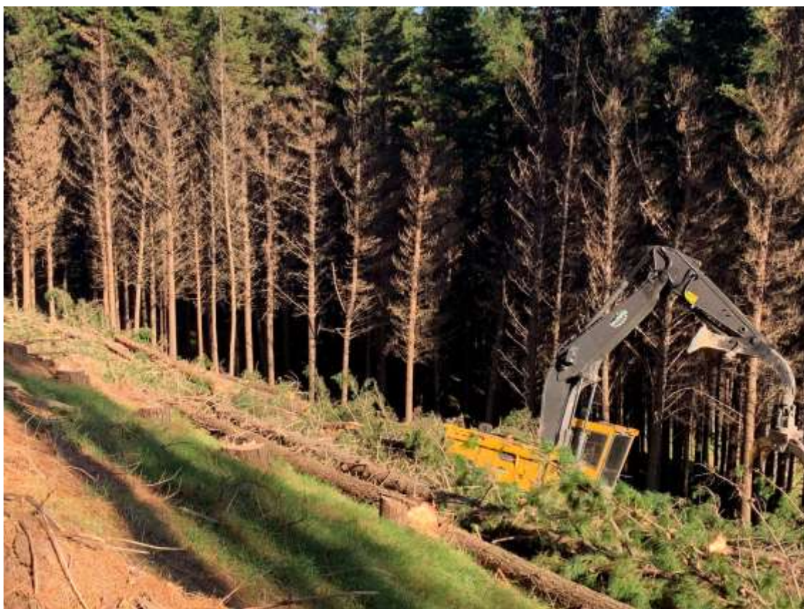
Photo 1: Log 16 working in Setting 501.
