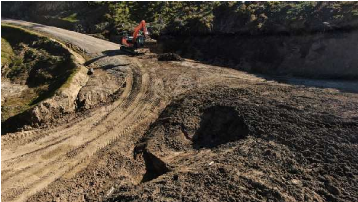
Photo 2: Setting 500, maintenance machine unblocking a culvert on Chrisdon Road after March storm events.
