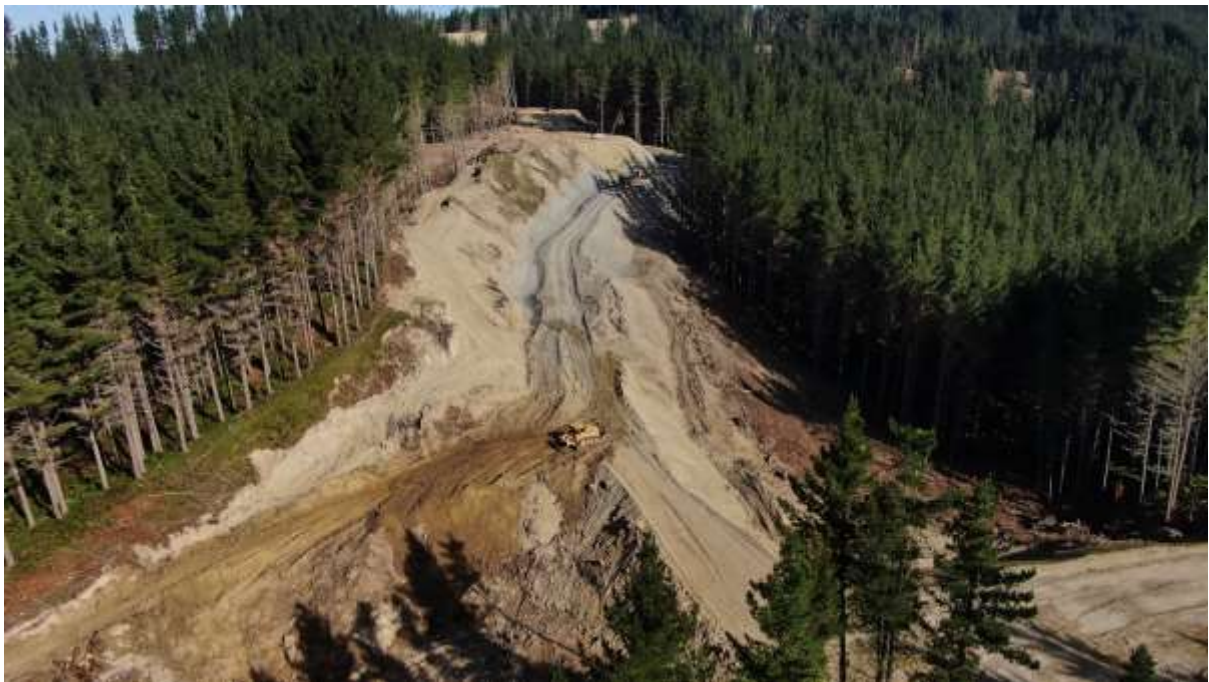
Photo 2: Earthworks crew forming Wah Road from Landing 17 to 18, Setting 506.
