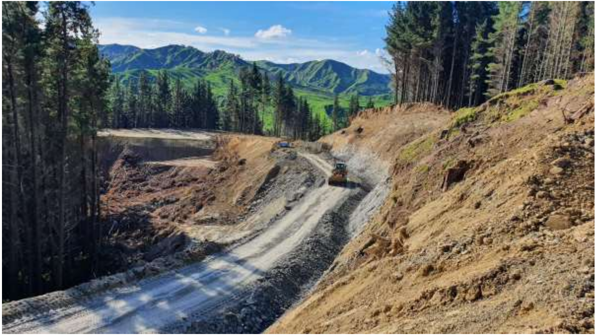
Photo 1: Earthworks crew forming Wah Road, Setting 506.
