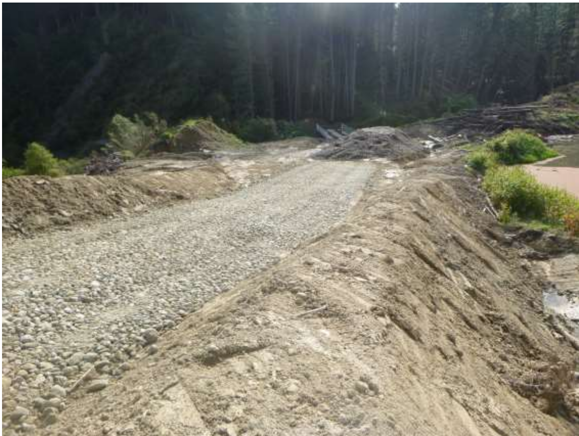
Photo 2: George Road bridge being metalled and post-harvest rehabilitation.
