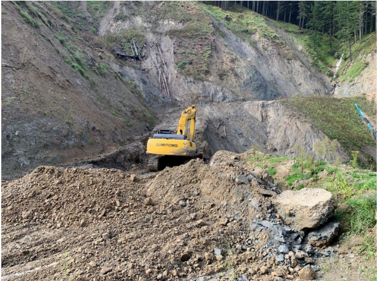
Photo 1: Sumitomo 370 working on large dropout at Marker 3 on Richmond Road.
