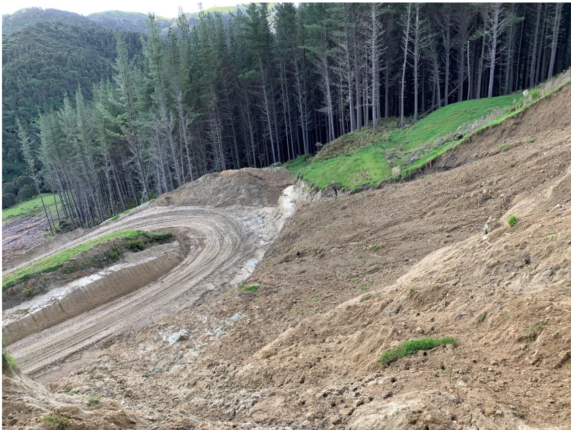
Photos 5 & 6: Large slip at G4 marker on Maloy Road.
