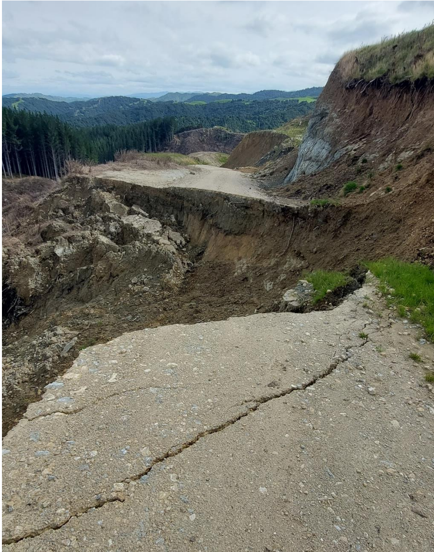
Photo 4: Large dropout on Cardiff Road.
