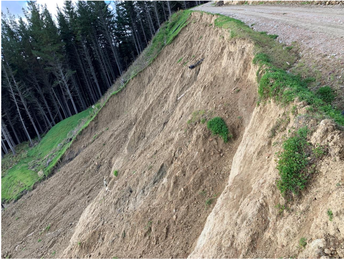
Photos 5 & 6: Large slip at G4 marker on Maloy Road.
