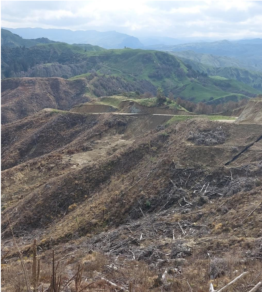
Photo 3: Large dropout on Cardiff Road.
