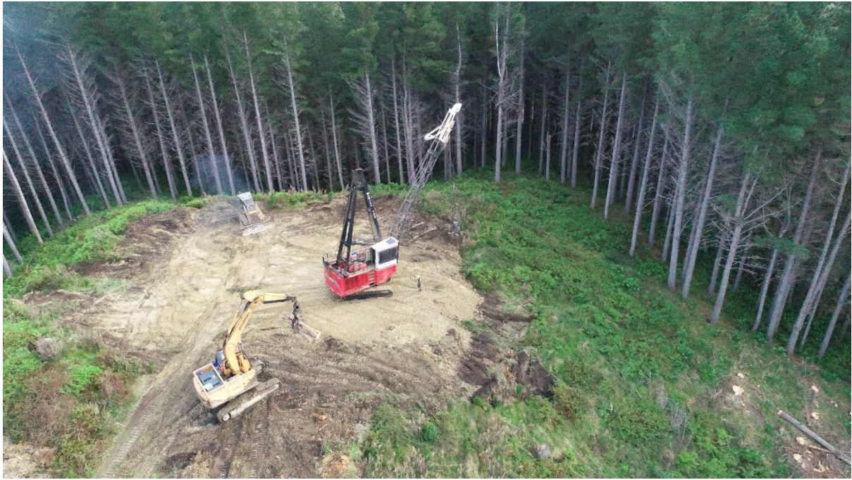
Photo 1: Positioning the swing yarder on Pad 27A before starting to pull the new area.
