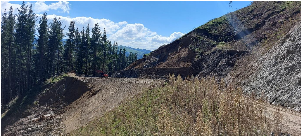
Photos 8, 9 & 10: Repaired dropout at Marker 3 on Richmond Road.
