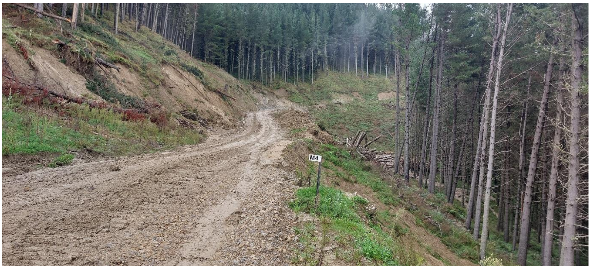
Photo 6: Marker 4, Richmond Road open again after a large slip blocked the road.
