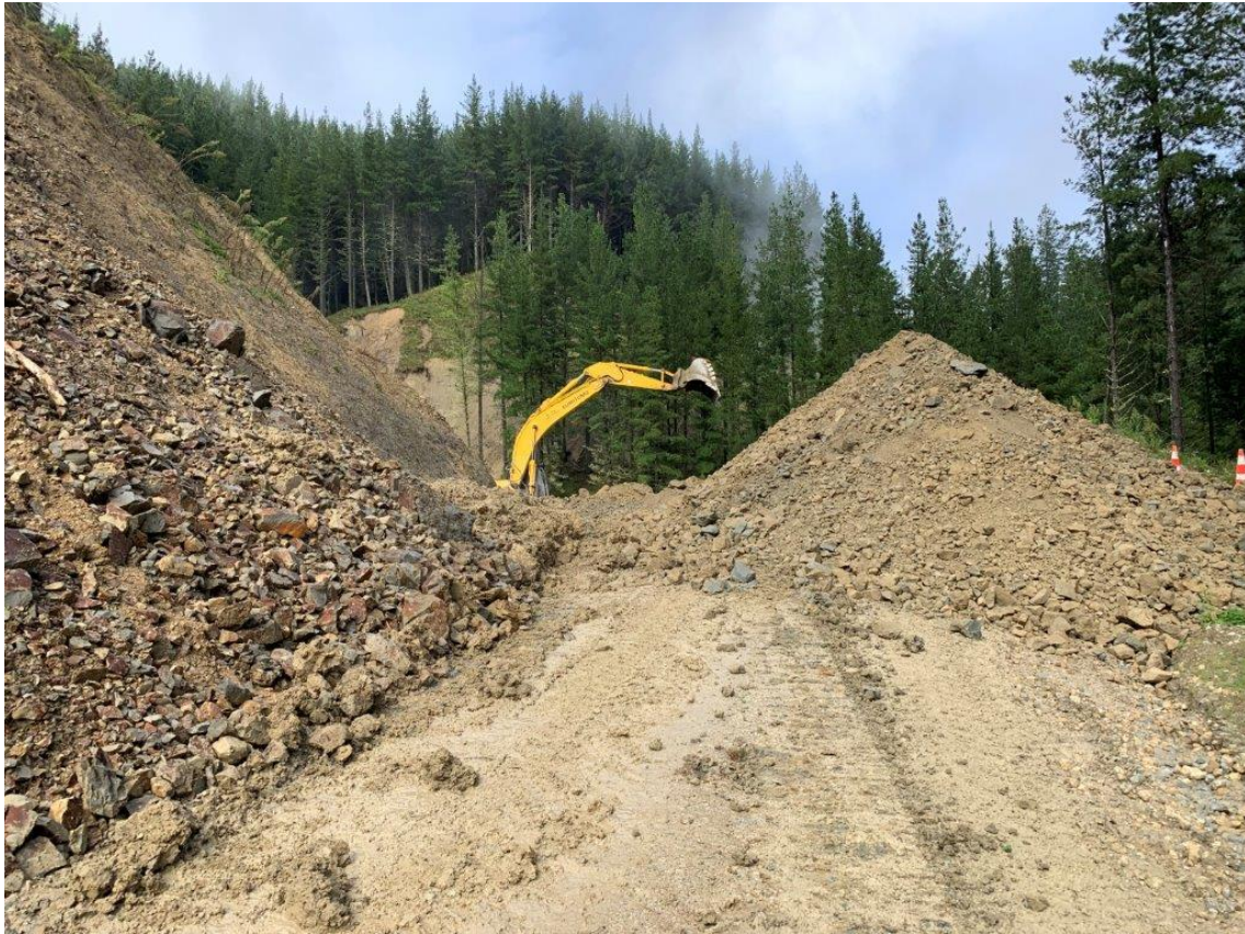
Photos 3 & 4: Sumitomo 370 working on large dropout at Marker 3 on Richmond Road.
