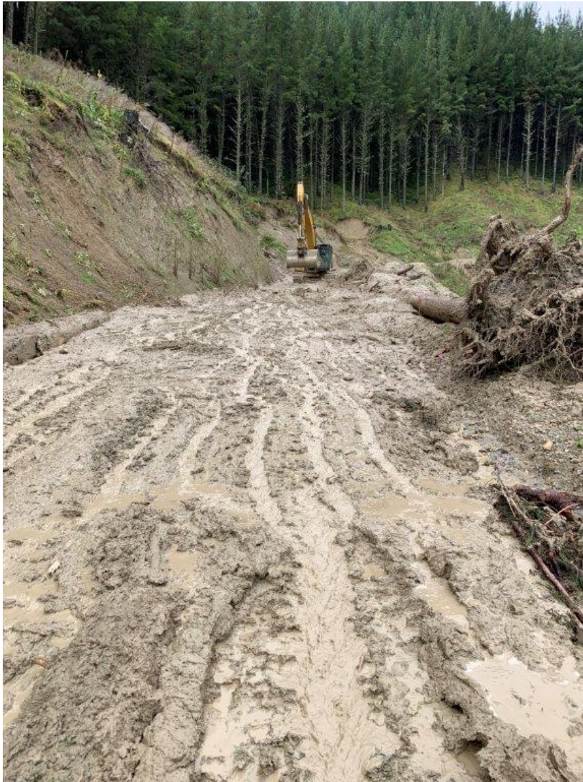
Photo 1: CAT 330 working on large slip at Marker 4 on Richmond Road.
