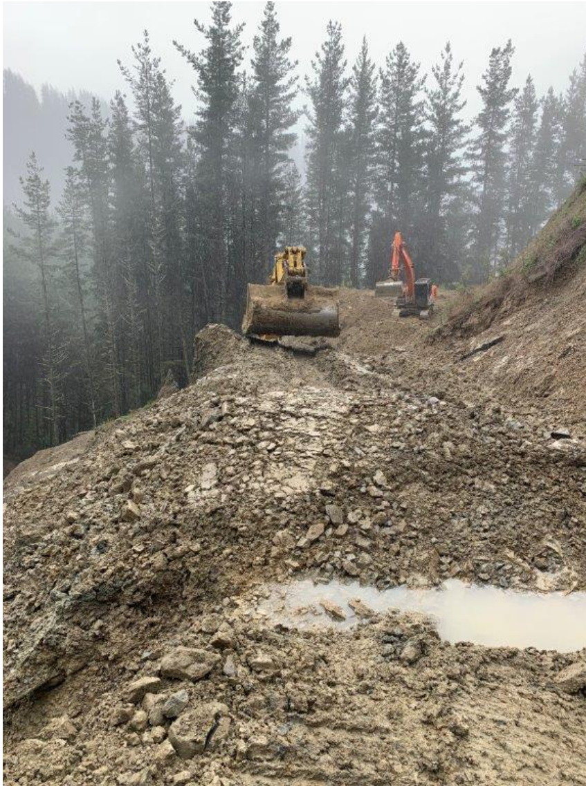
Photo 2: Tahurua Earthmovers starting repair on large dropout between Marker 3 and 4 on Richmond Road.
