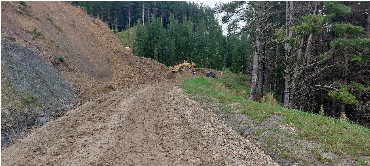
Photo 5: CAT D8 working on Richmond Road dropout.
