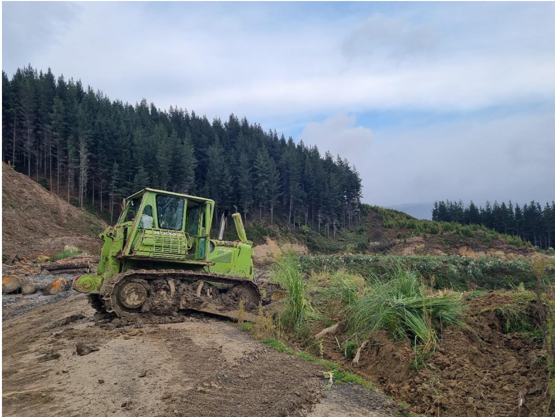
Photo 1: Old T-rex bulldozer being used as the backline anchor machine for the hauler.
