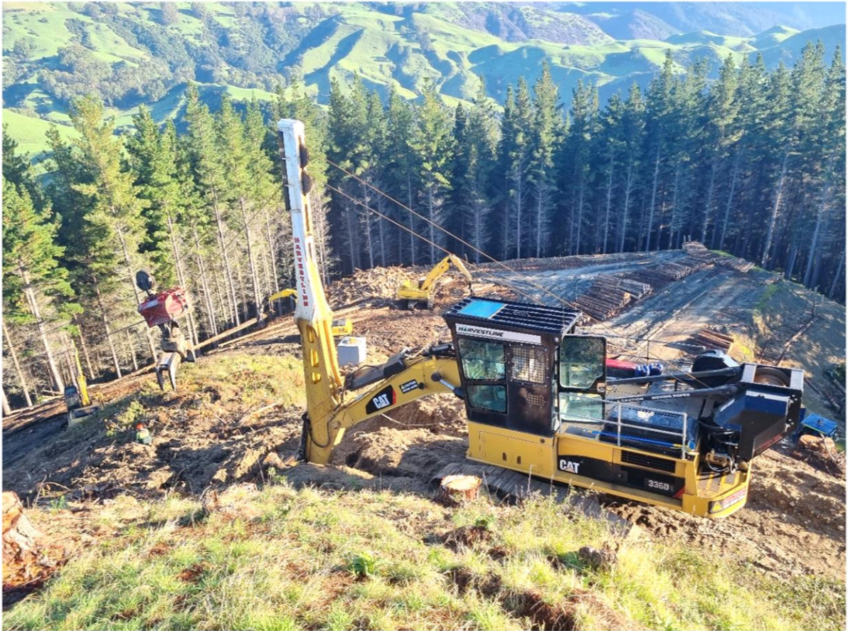
Looking down at harvestline machine on Pad 144A with Landing 144 in background.
