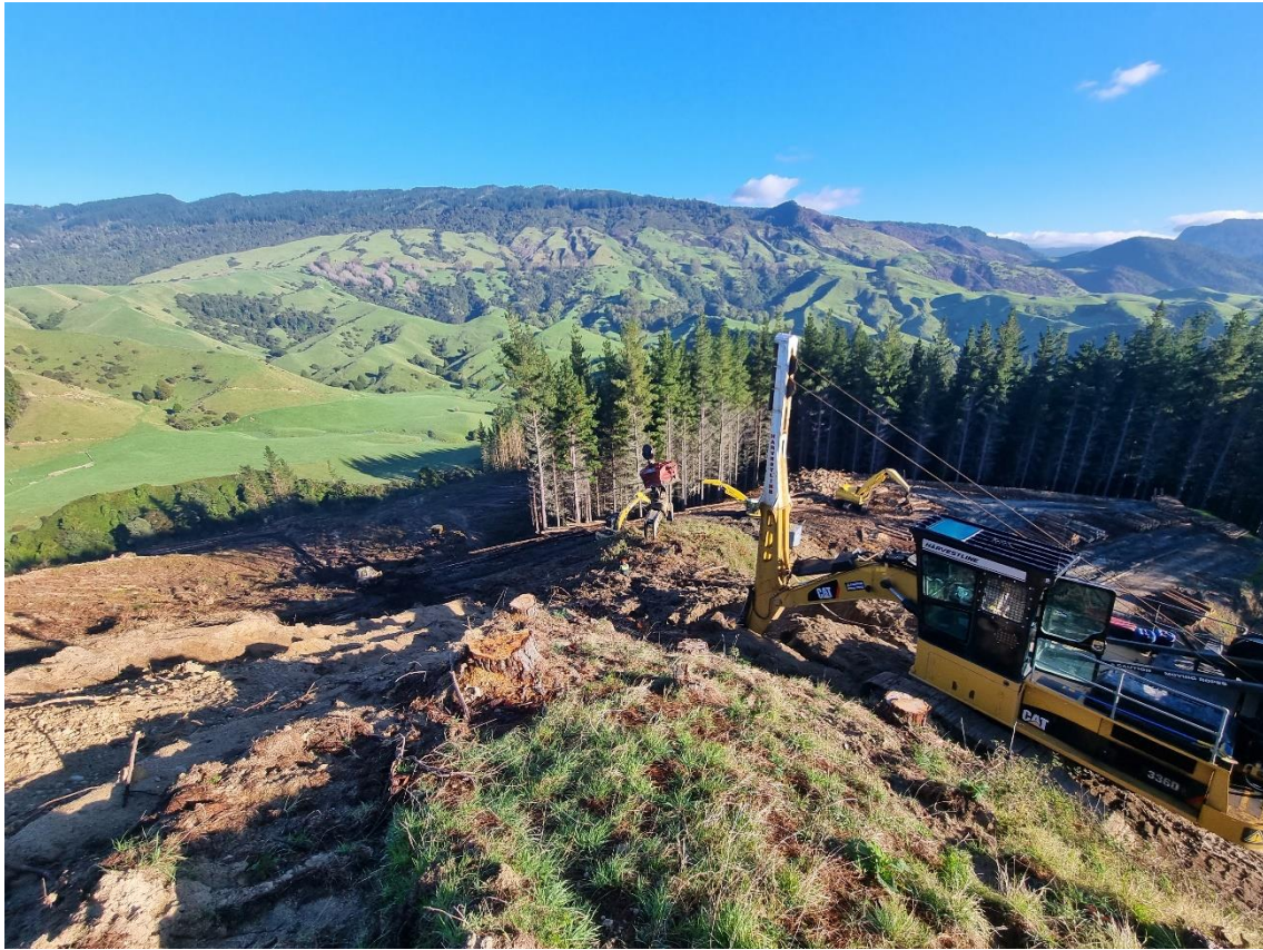
Photo 1: Looking down the haul corridor into Setting 144.
