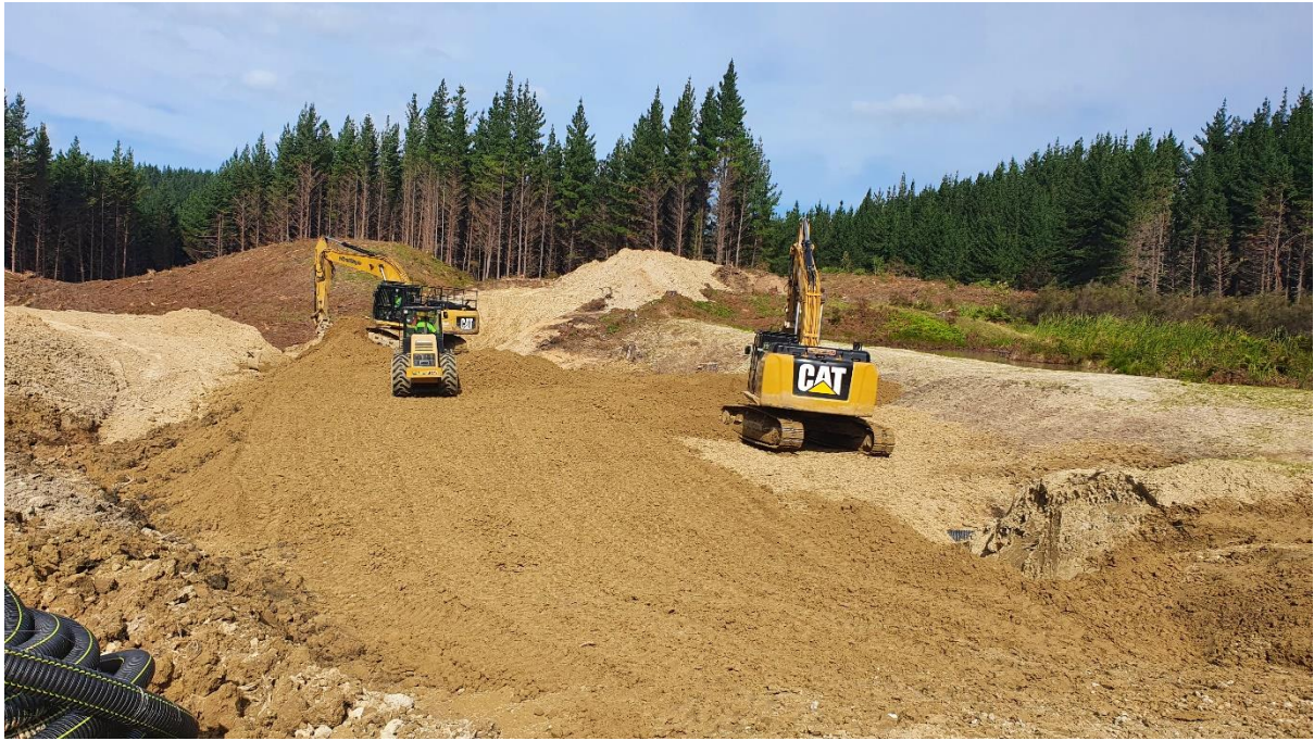
Photo 3: Earthworks almost ready for pavement, Chrisdon Road.
