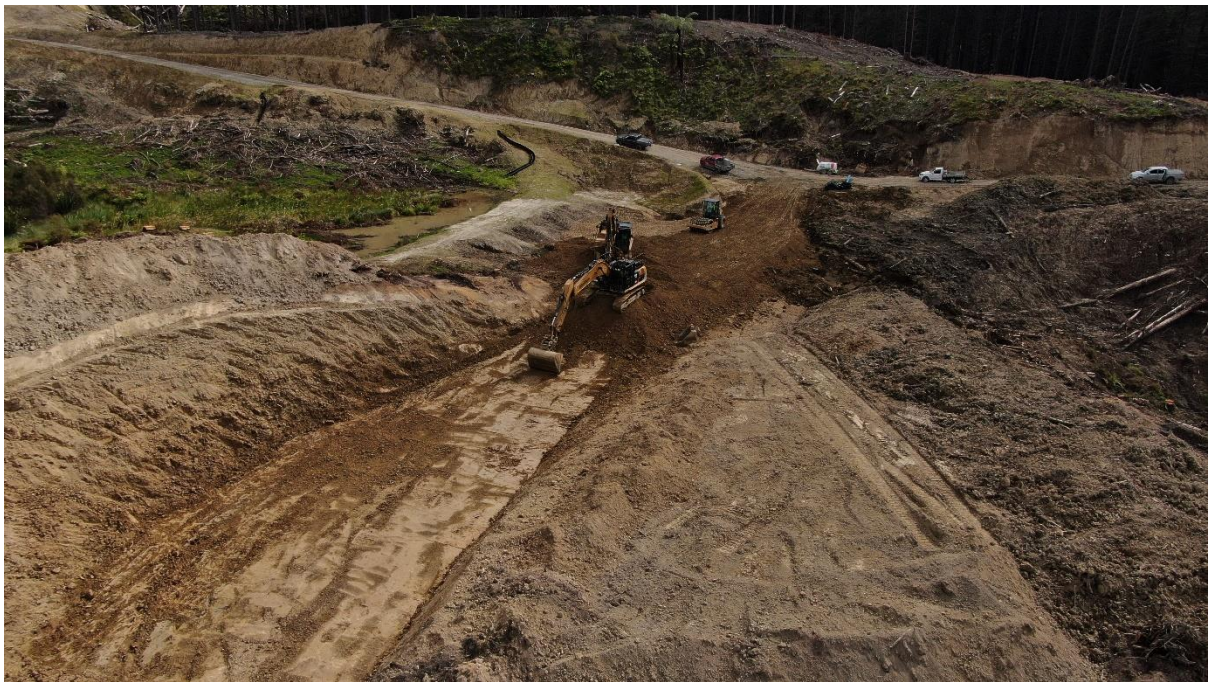
Photo 2: Crew undertaking roading below dam wall on Chrisdon Road, Setting 500.
