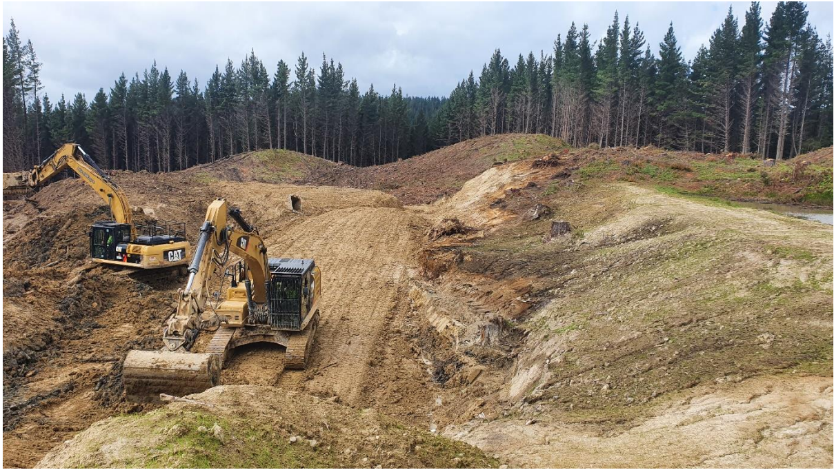
Photo 1: Crew undertaking earthworks for road crossing below wetland in Setting 500.
