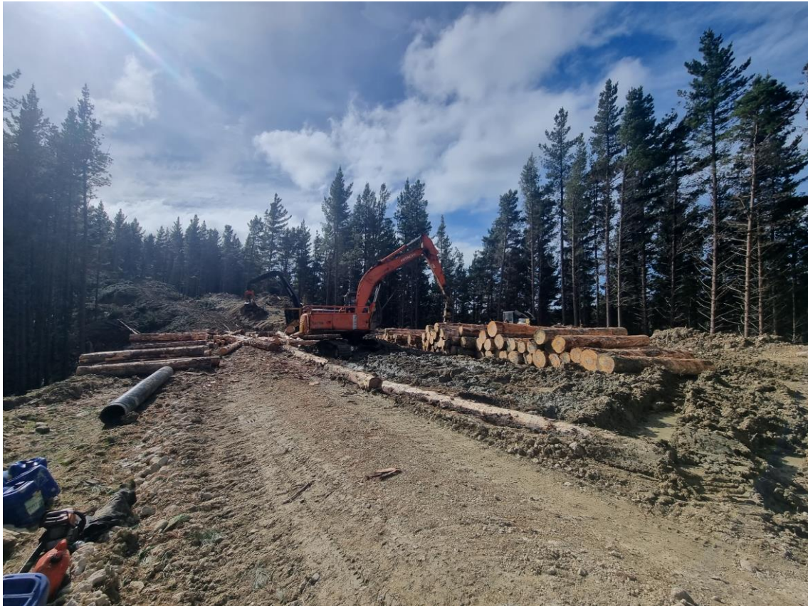
Photo 1: loader sorting logs into stacks on Landing 39.
