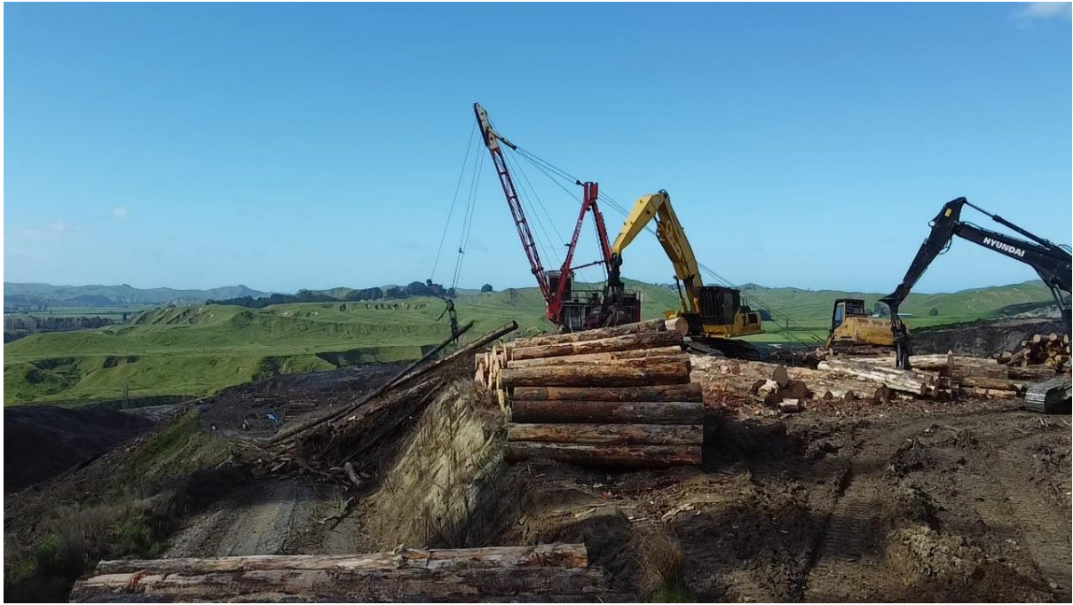
Photo 5: Setting 18 - Swing yarder pulling stems over road to Pad 18A.
