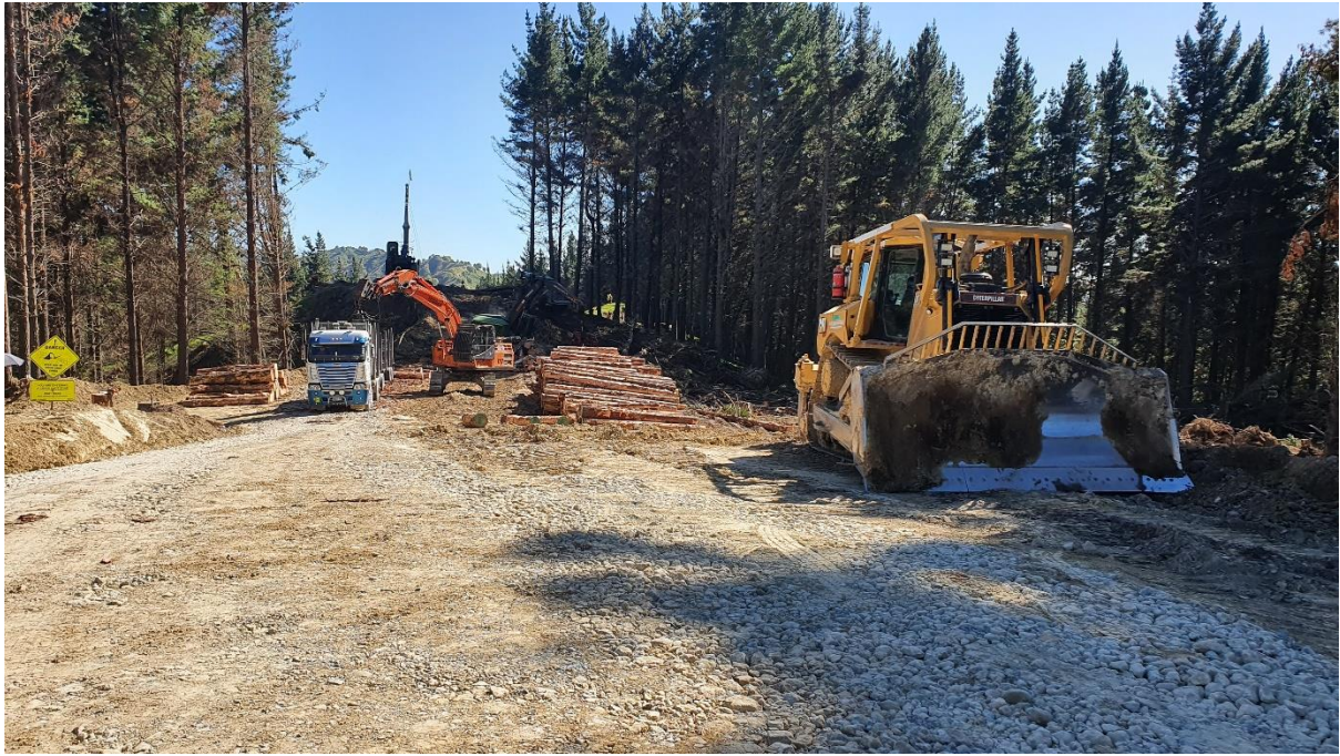
Photo 1: Loading truck on Landing 17, roadlining Setting 506 on the boundary of Castle Rock and Hunter Valley Forests.
