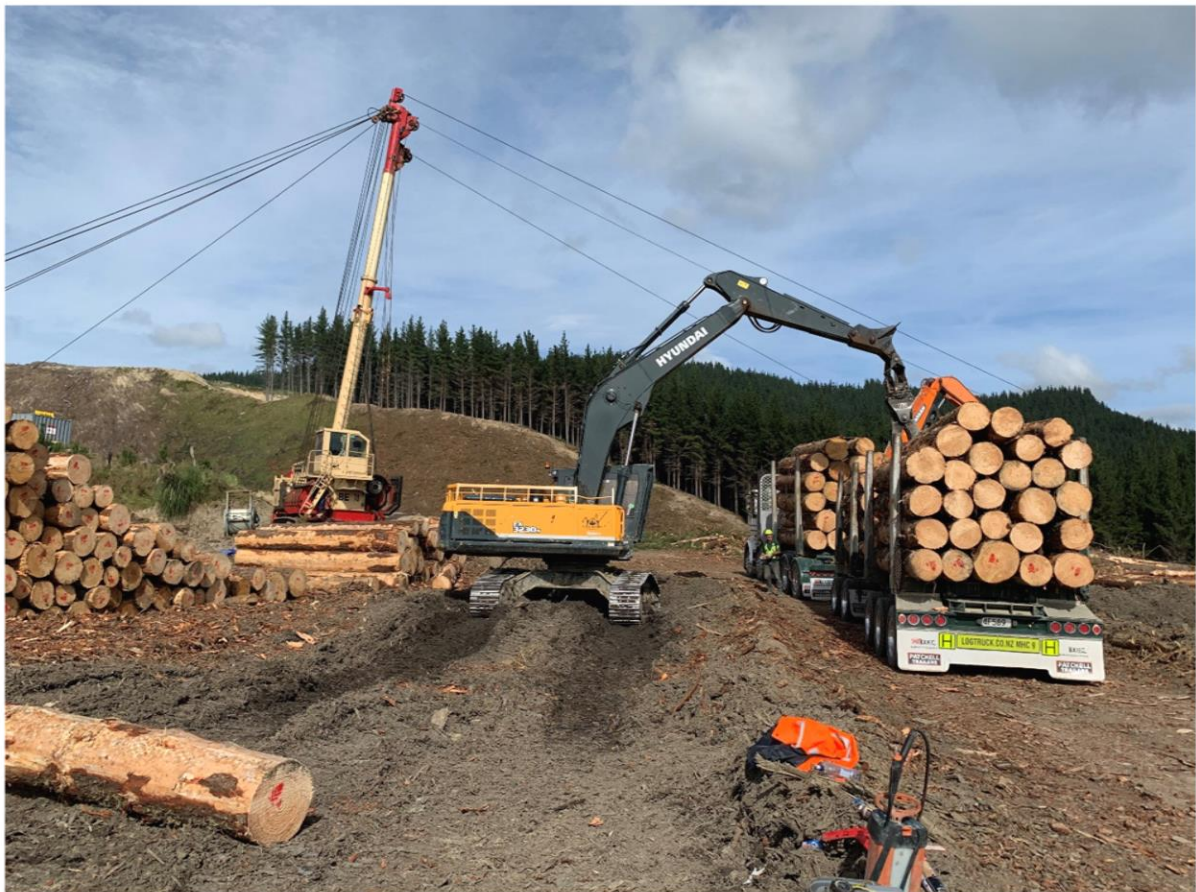
Hauler pulling the last of Setting 7 in Hunters Road while a truck is being loaded.
