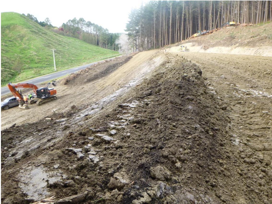
Photos 7 & 8: Entrance into Mad Mutt Road being formed by Tahurua Earthmovers.
