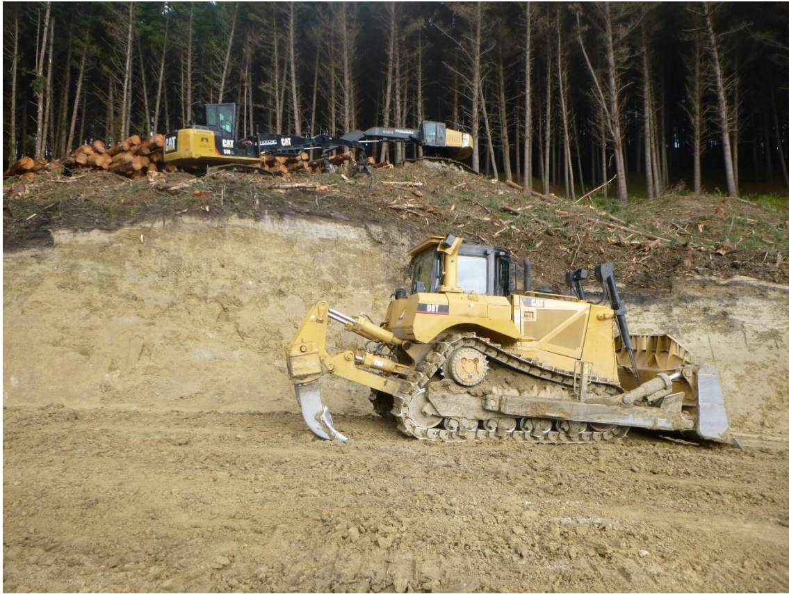
Photo 9: Landing 1 formation by Tahurua Earthmovers.
