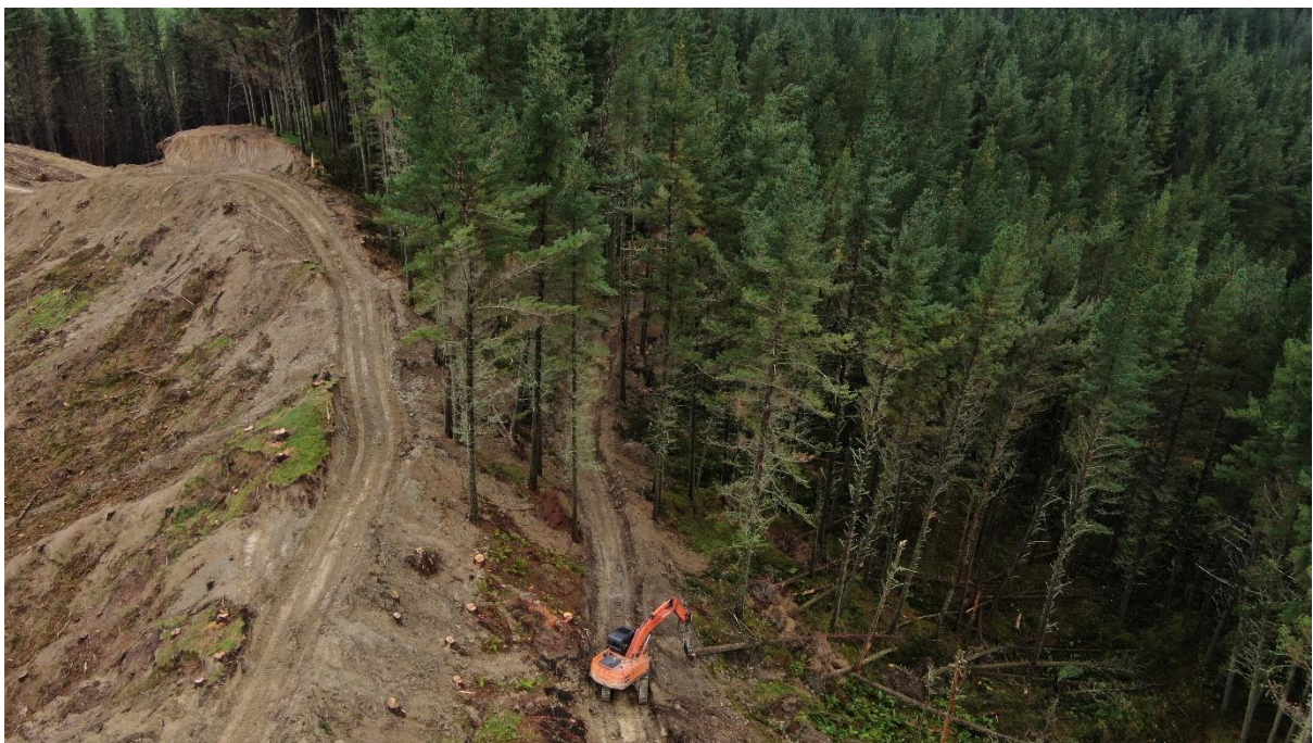
Photo 2: Setting 506 roadlining area for earthworks crew to undertake works.
