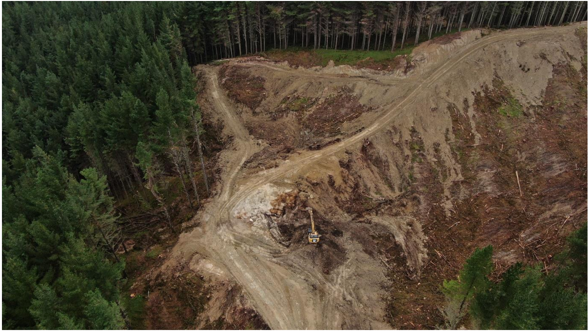
Photo 3: Setting 506, earthworks crew forming Landing 18.
