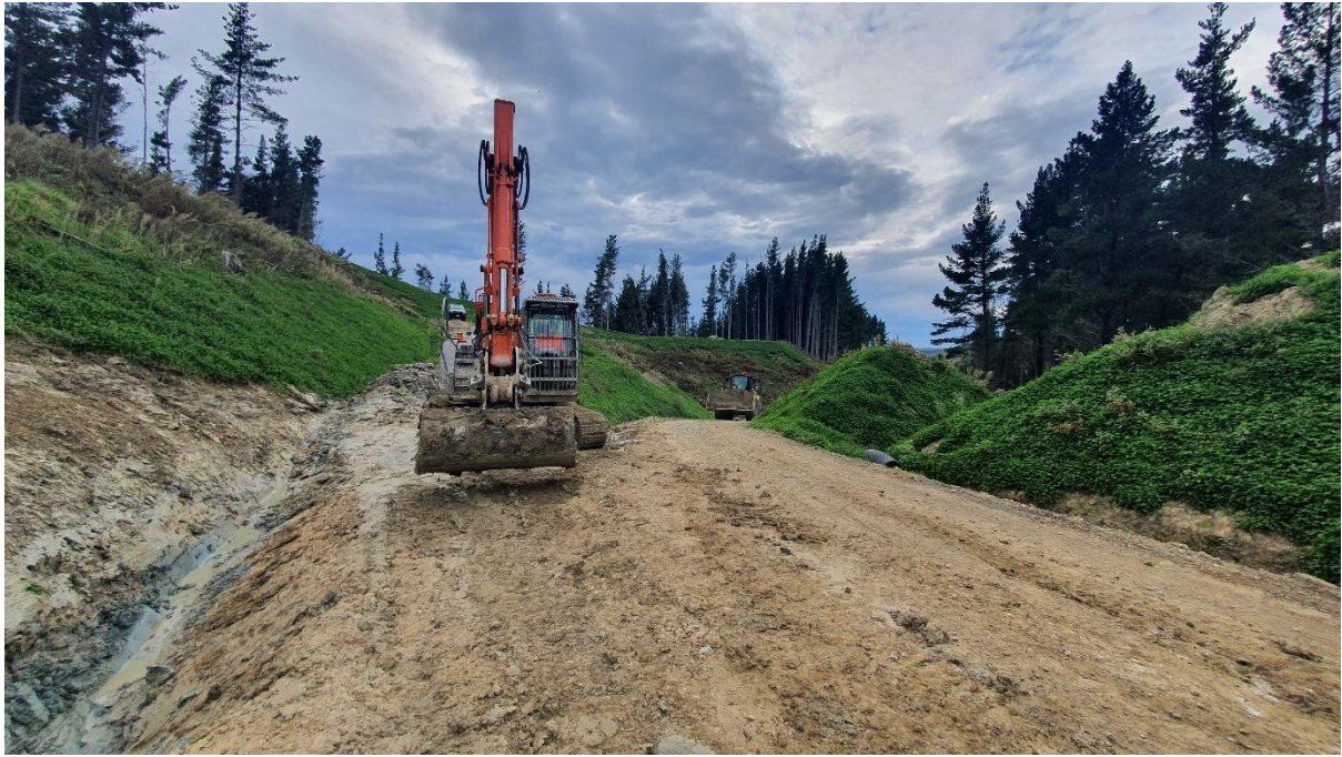
Photo 1: Maintenance crews in forest opening roads after storm events.
