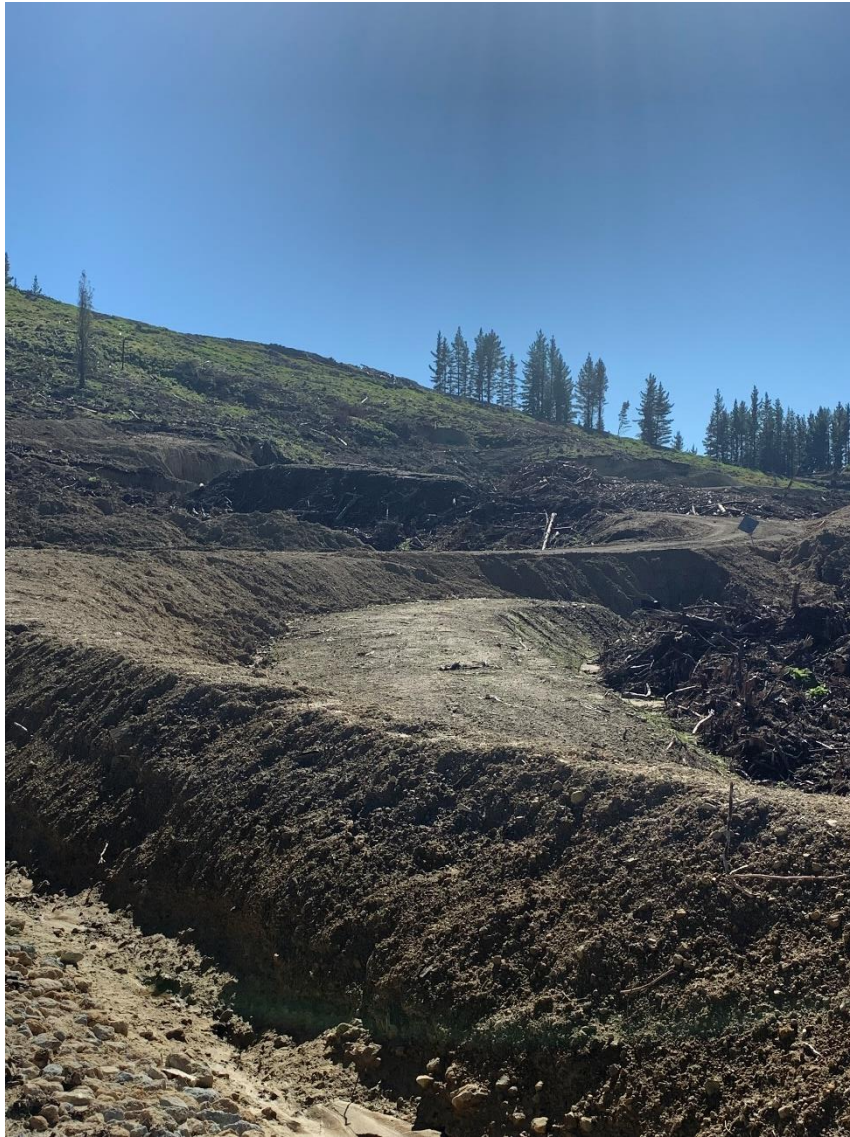
Photo 6: Section of road between Landings 914 and 915.
