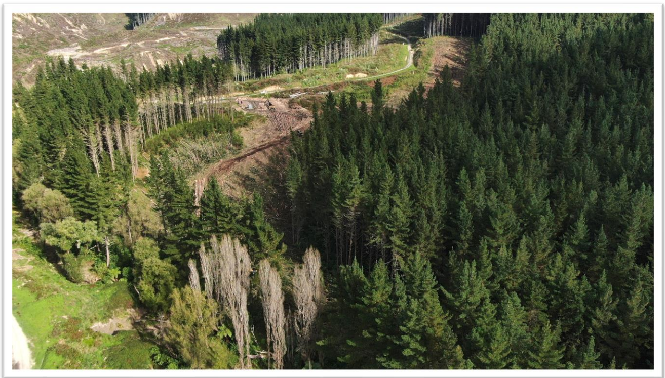
Aerial image of Setting 9 progress.
