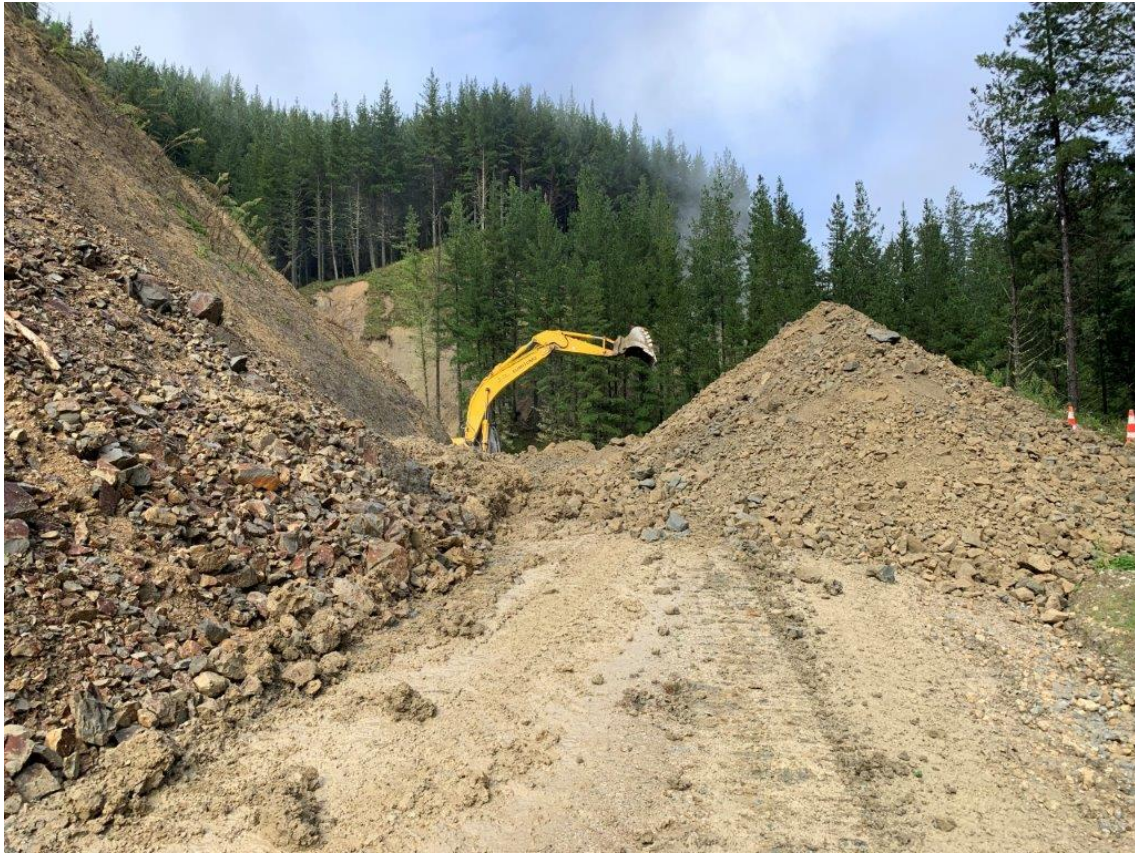
Photos 1 & 2: Sumitomo 370 working on large dropout at Marker 3 on Richmond Road.
