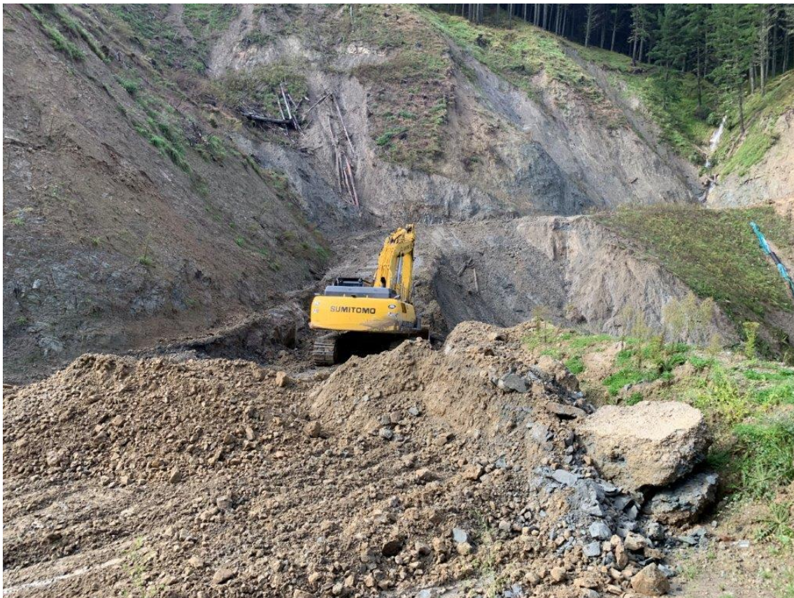
Photos 1 & 2: Sumitomo 370 working on large dropout at Marker 3 on Richmond Road.
