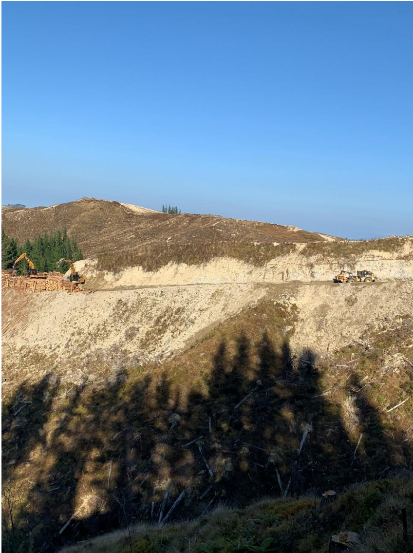
Photo 5: Log 28 working in Setting 605.
