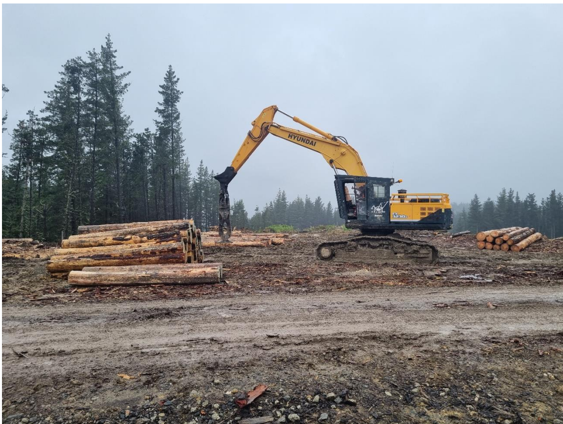
Photo 4: Loader machine stacking logs.
