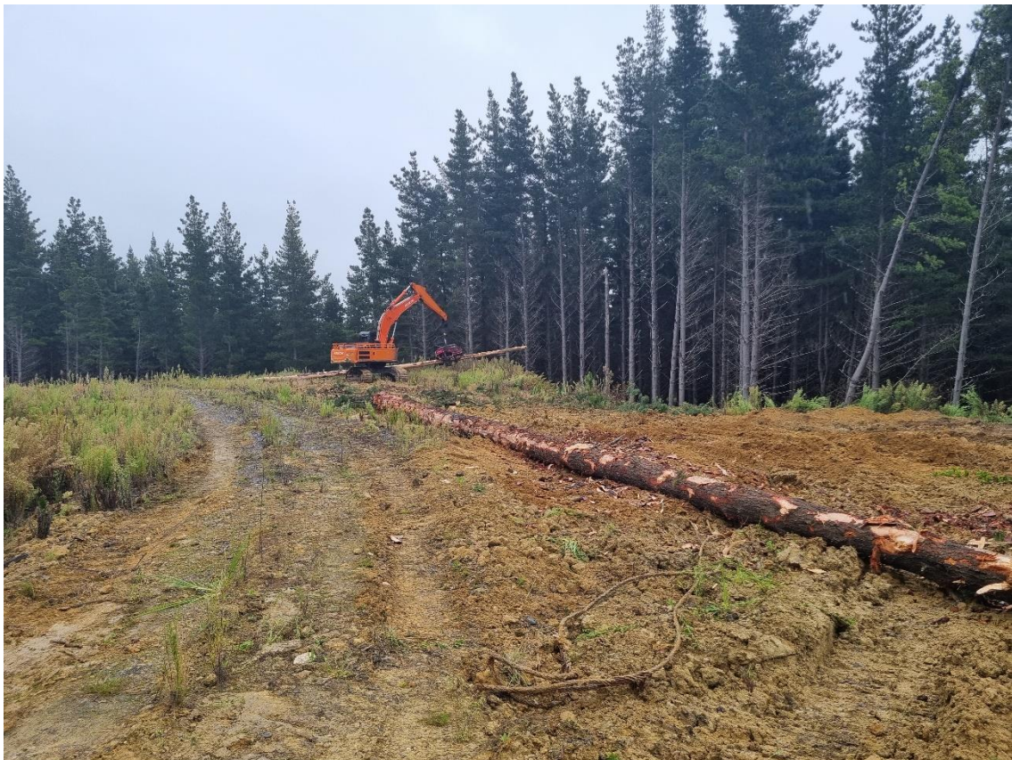
Photo 8: Processor machine working out his processing circle.
