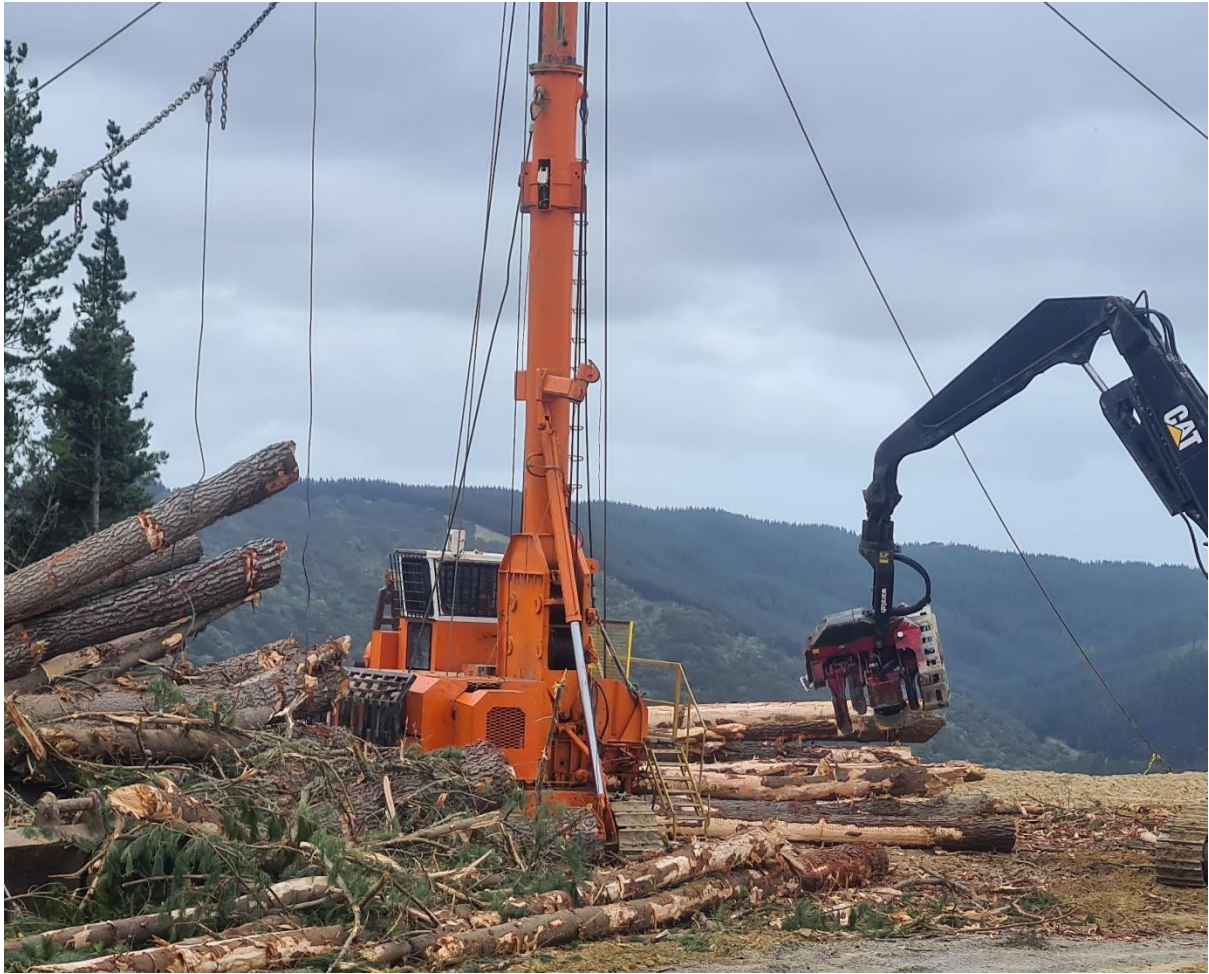
Photo 3: Swing yarder at work on Setting 8.
