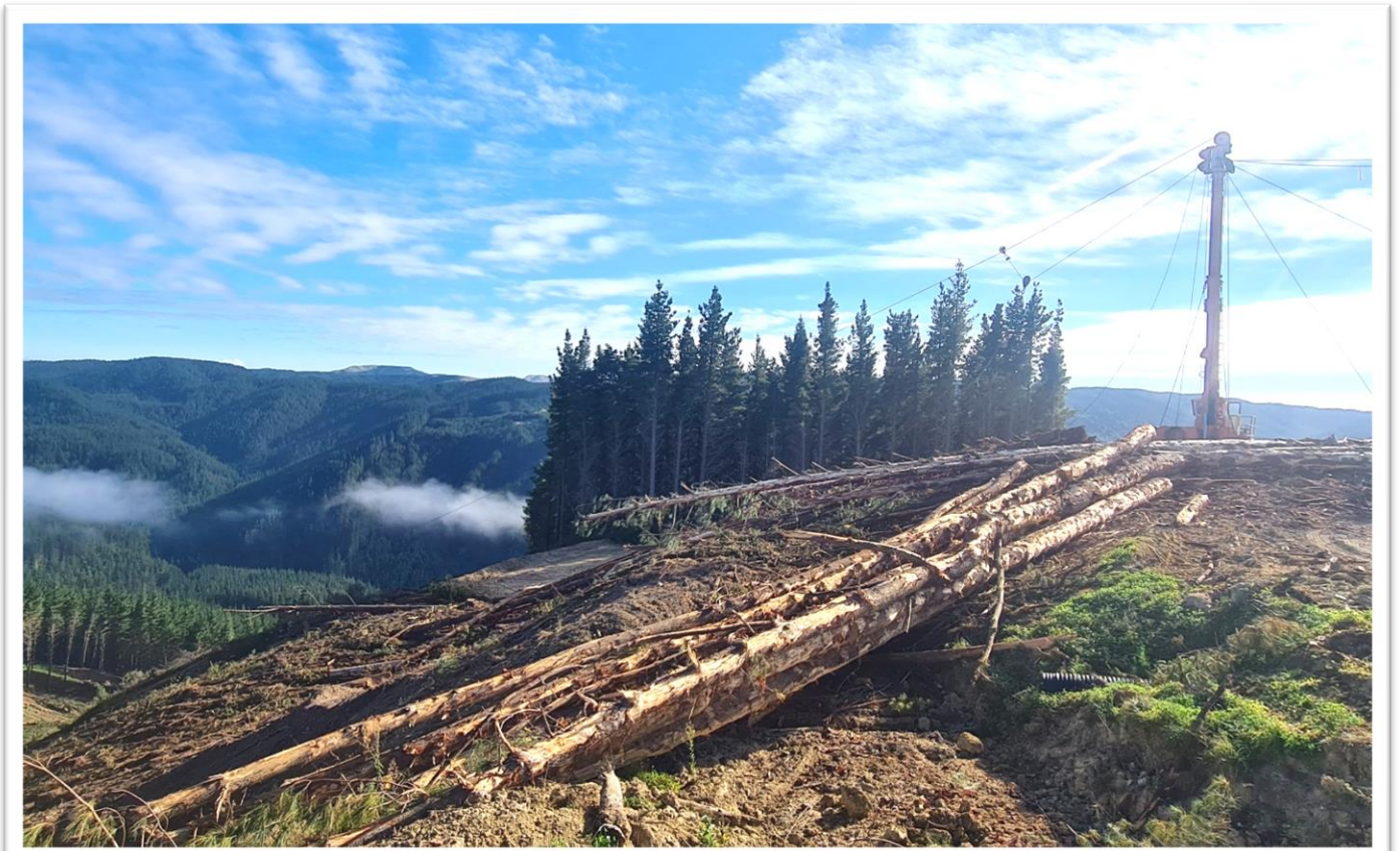
Yarder set up on Landing 8.
