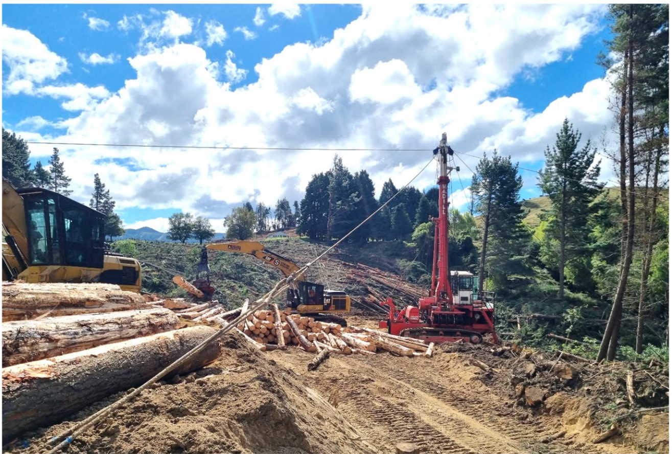
Looking back at the Madill 171 machine along the guy rope.
