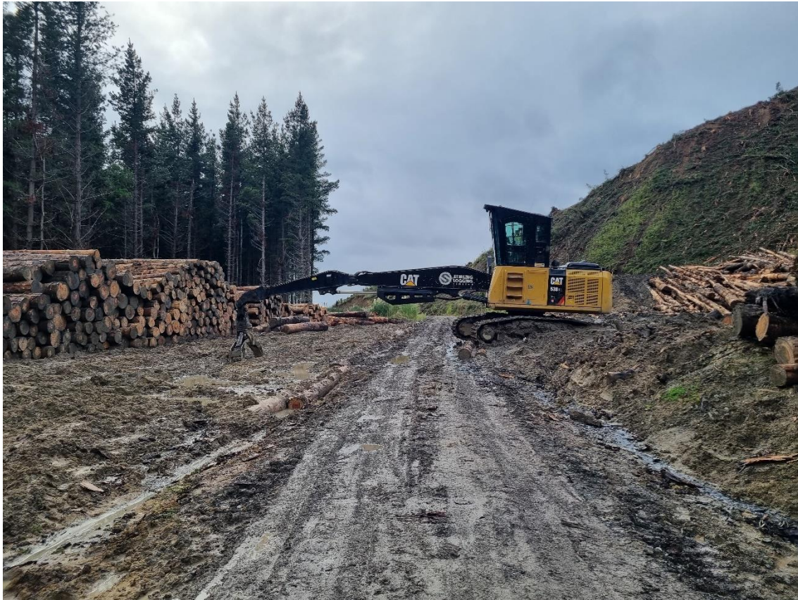
Photo 1: Loader machine on Landing 103.
