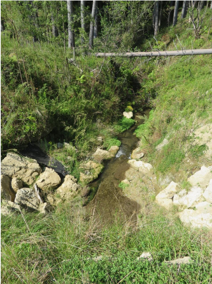
Photo 1: Standing on 2400 mm culvert crossing looking at retained gravel in stream bed.
