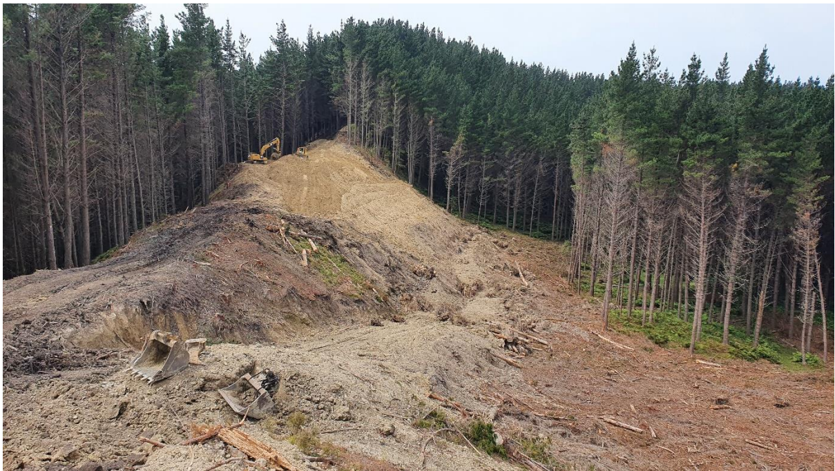
Photo 2: Roadline Setting 500, earthworks crew working on Landing 23.
