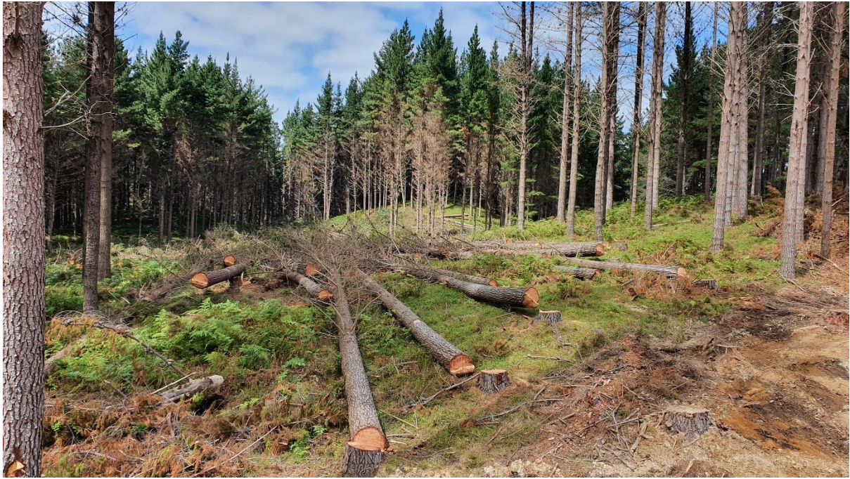
Photo 1: Commencing roadline in Setting 504, Chrisdon Road, Landing 19.
