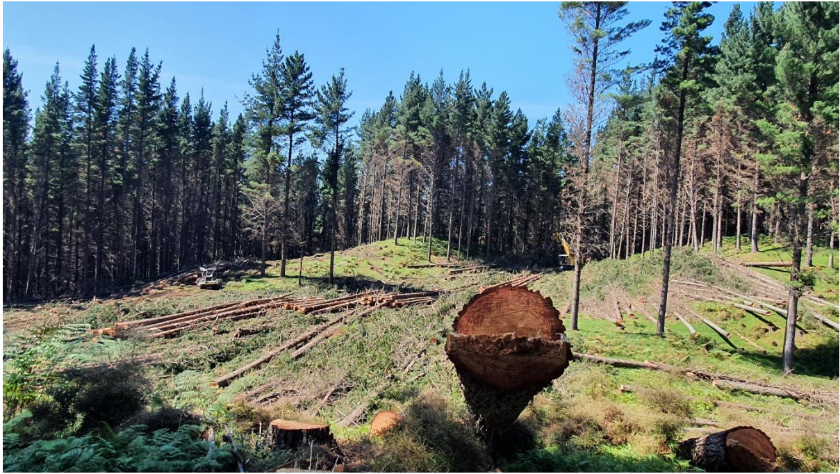
Photo 5: Opening up area for Chrisdon Road.
