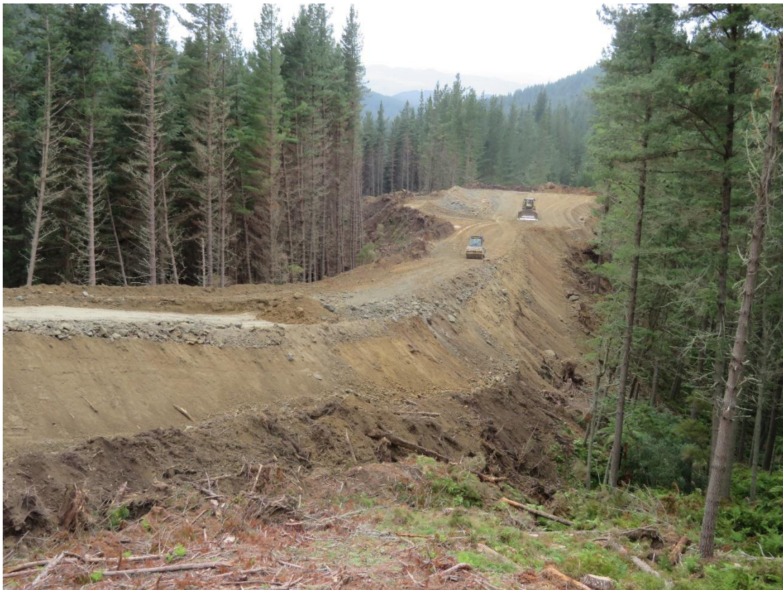
Photo 3: Road construction on Landing 122, Gleeson Road.
