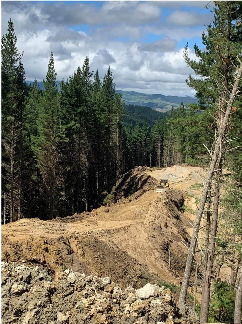
Photo 1: Tahurua Earthmovers working on Gleeson Road.
