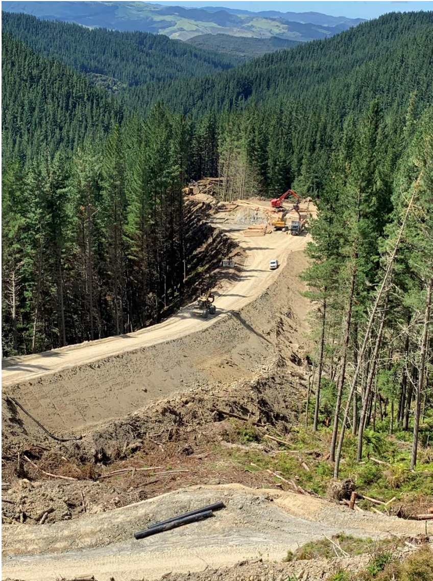
Photo 6: Log 16 working in roadline Setting 545, Gleeson Road.
