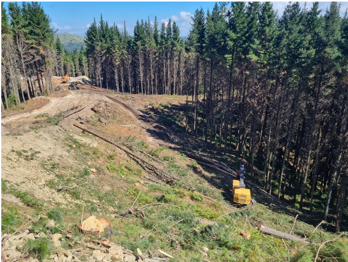
Photo 4: Roadline corridor extraction operation.
