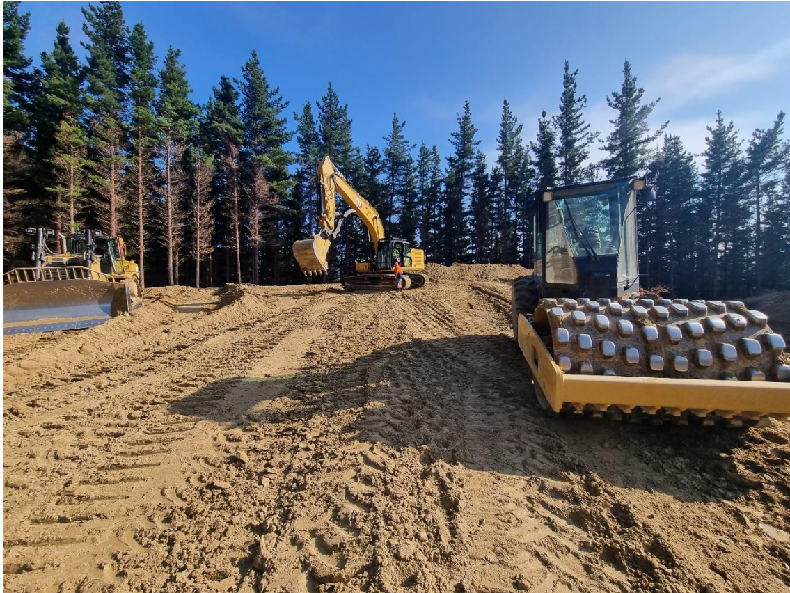
Photo 3: Landing under construction.
