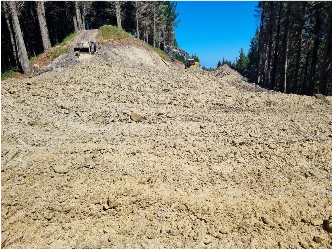
Photo 5: Formation of Landing 39 being carried out.
