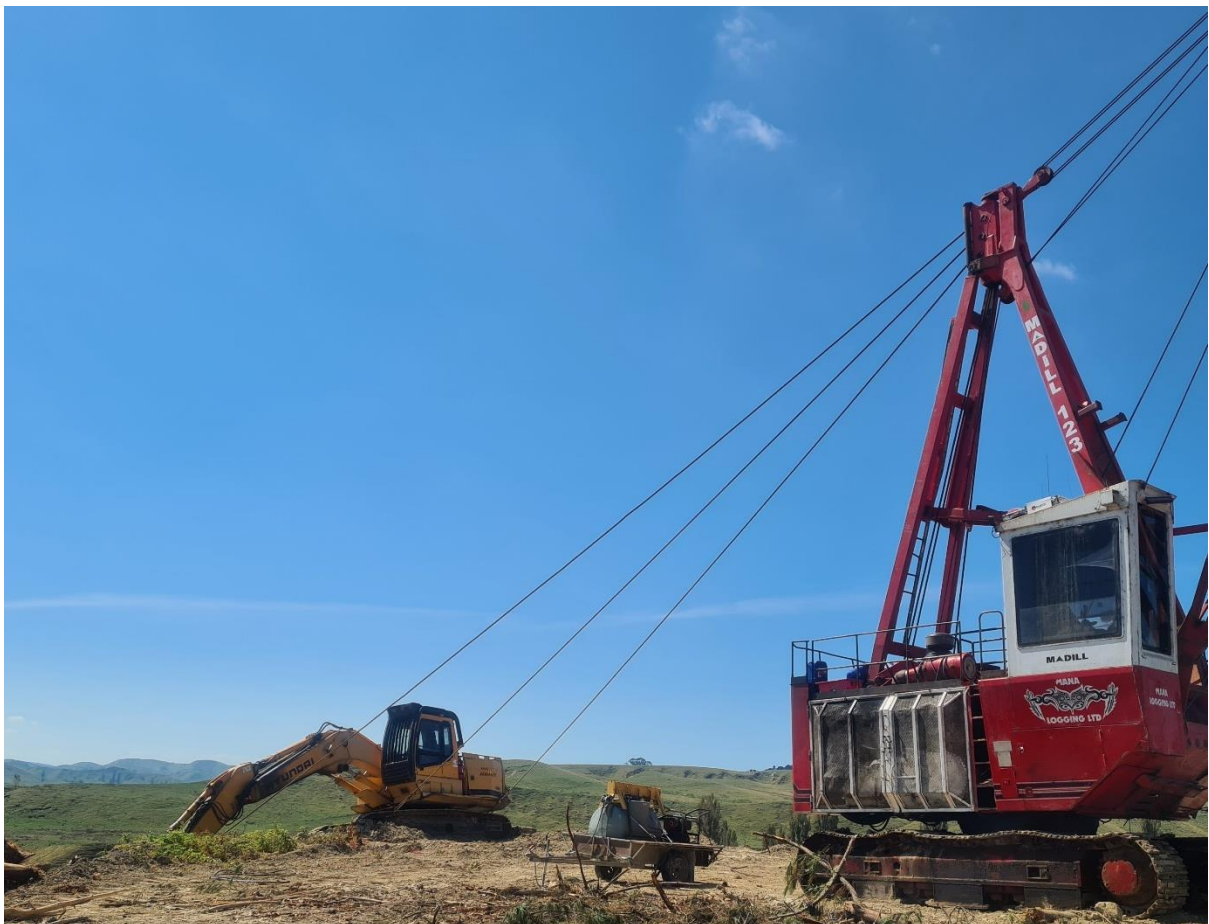
Photo 4: Digger being used as a deadman to anchor the hauler.
