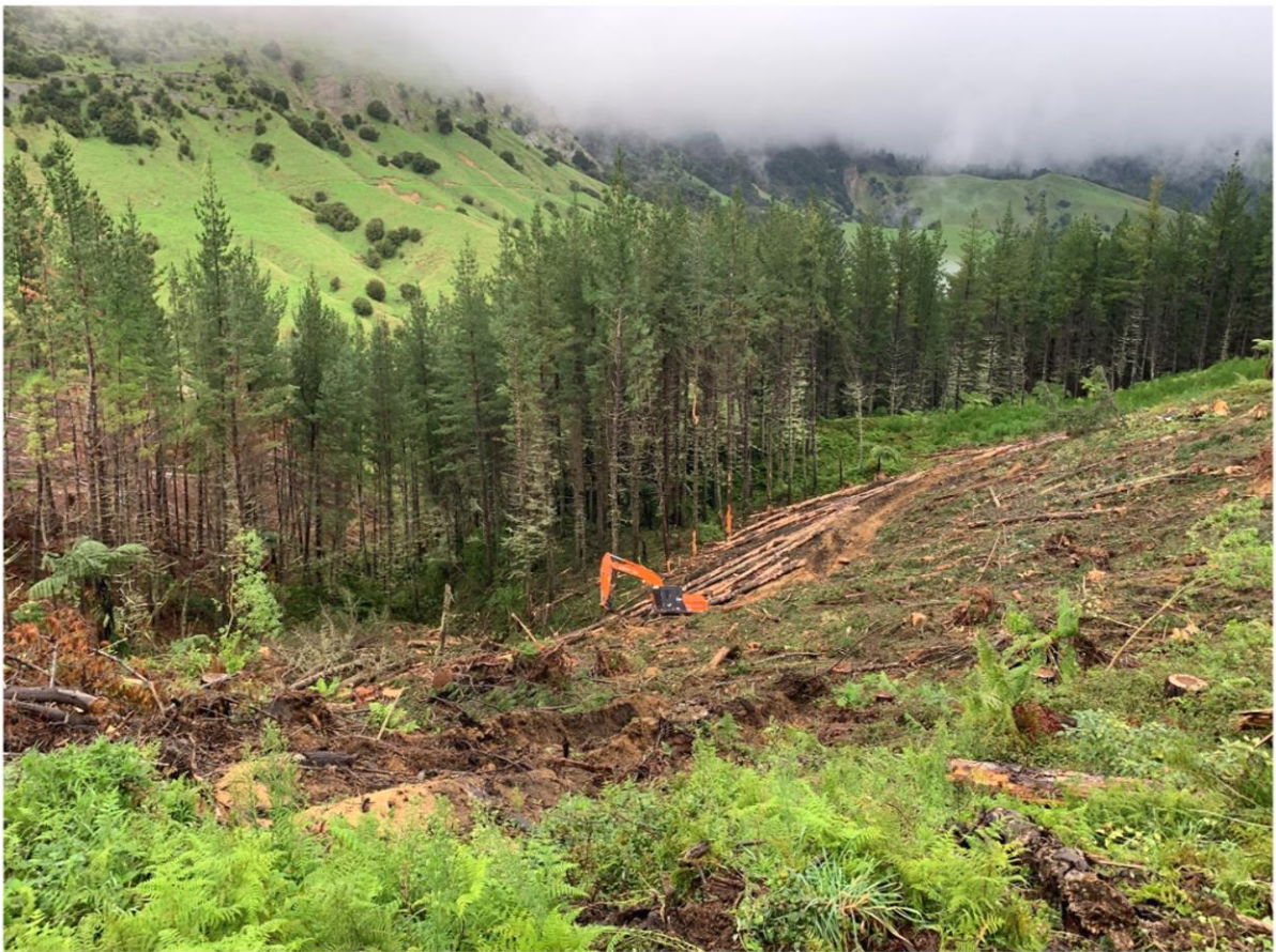
Shovelling the right hand side of Setting 69.
