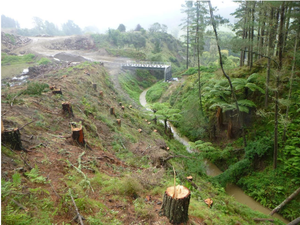
Photo 3: Bridge, Landing 4 and cutover in the background.
