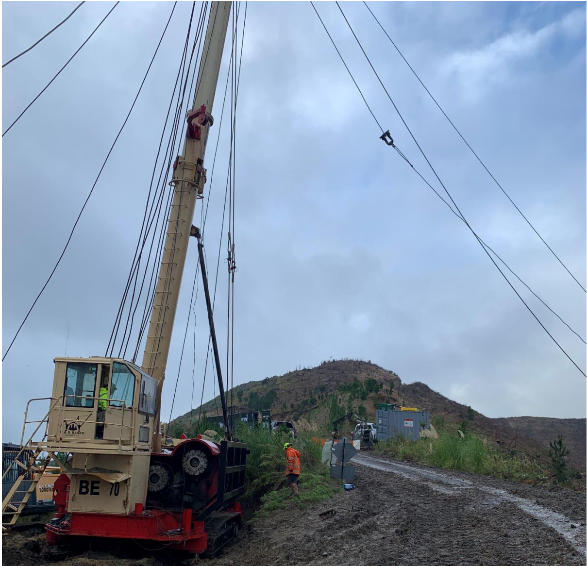
Photo 6: Shifting hauler to get deflection in setting.
