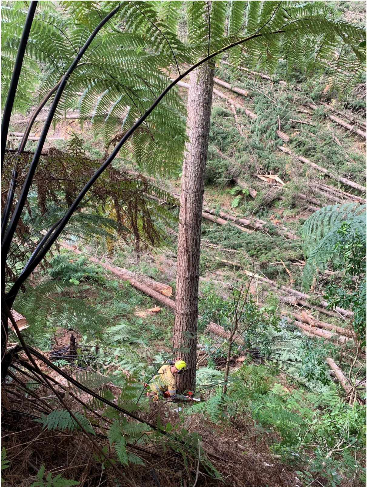
Photo 1: Faller hammering in a wedge before completing back-cut to fell tree.
