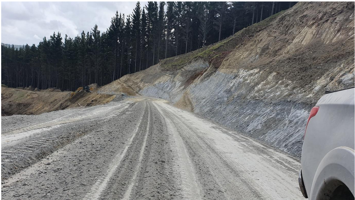
Photo 6: Roadline Setting 506, inspecting a near complete subgrade on Wah Road.
