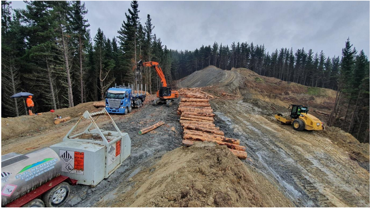
Photo 1: Setting 500, processing at Wah Road intersection.
