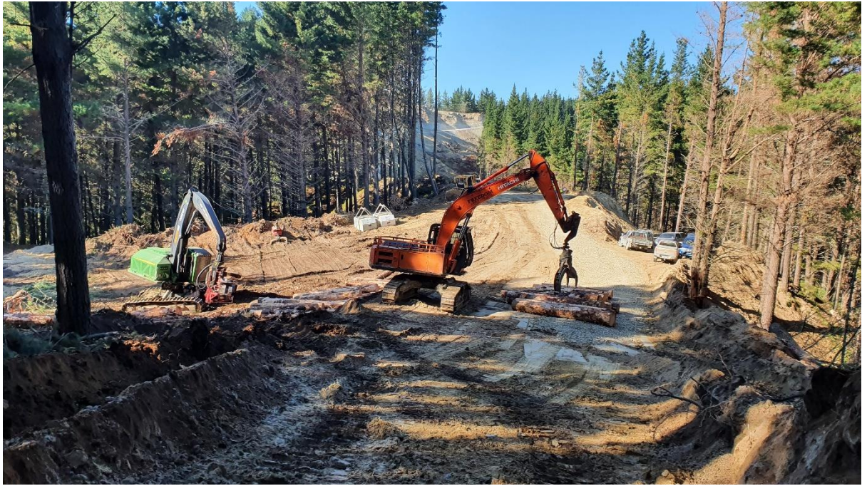
Photo 7: Roadline Setting 506, crew beginning processing at Landing 17.
