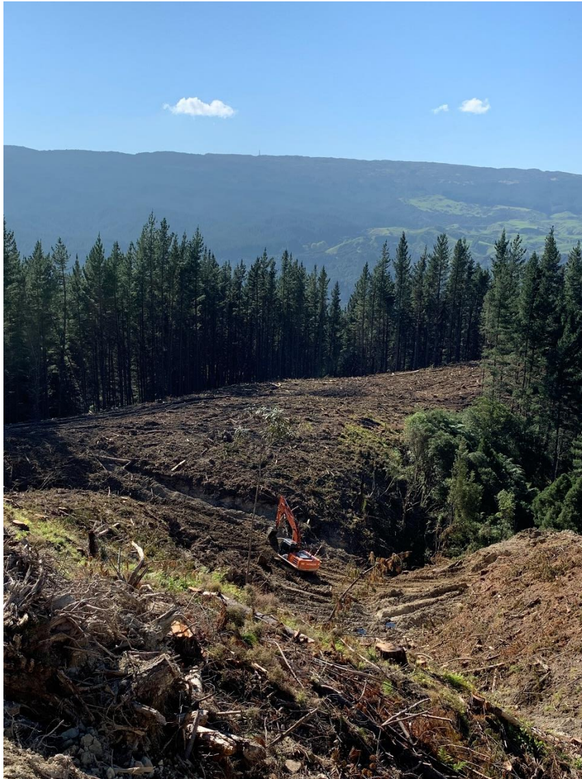
Photo 3: Tahurua Earthmovers building Bradley Road.
