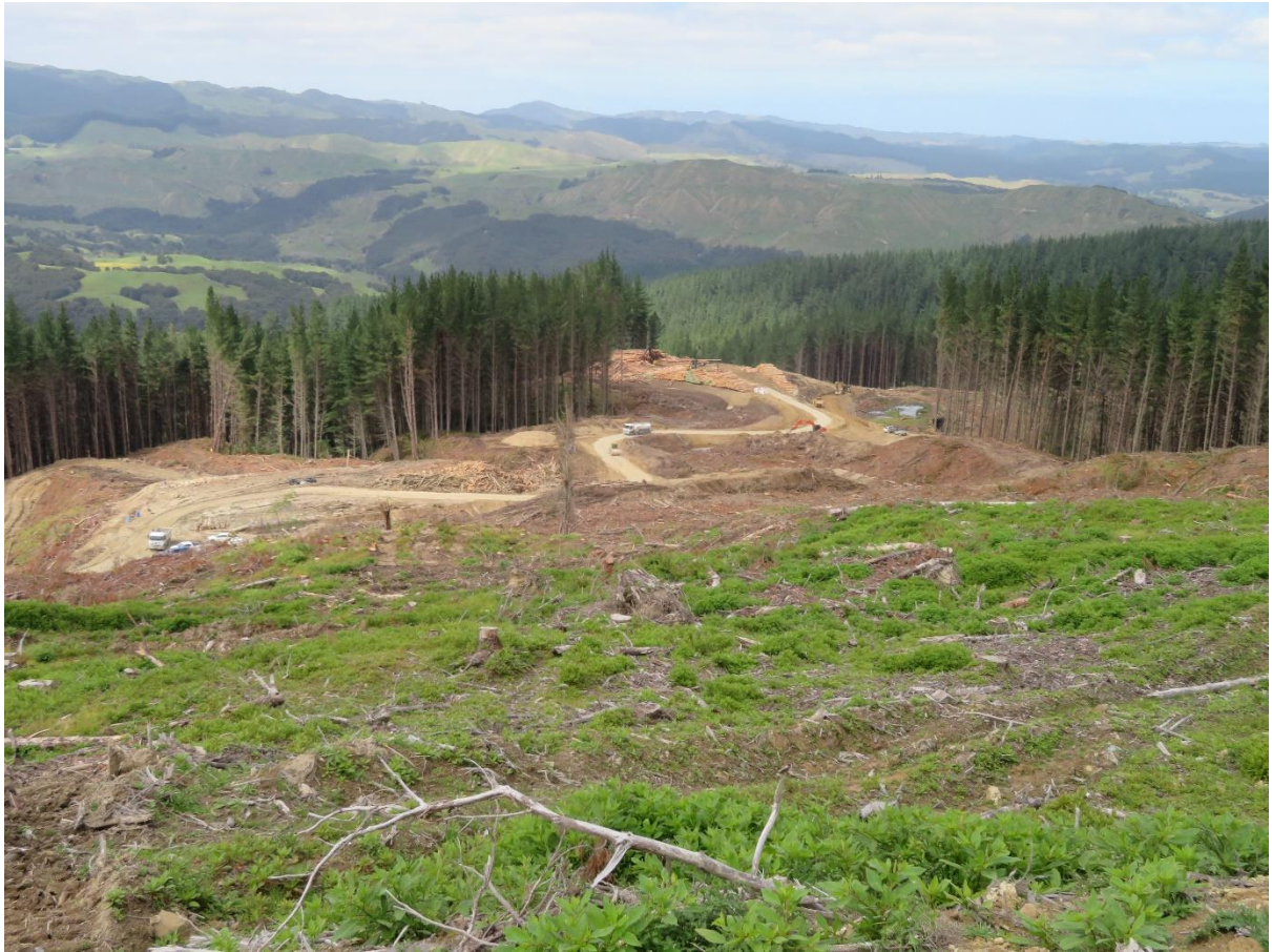
Photo 1: Road construction to Landing 914.
