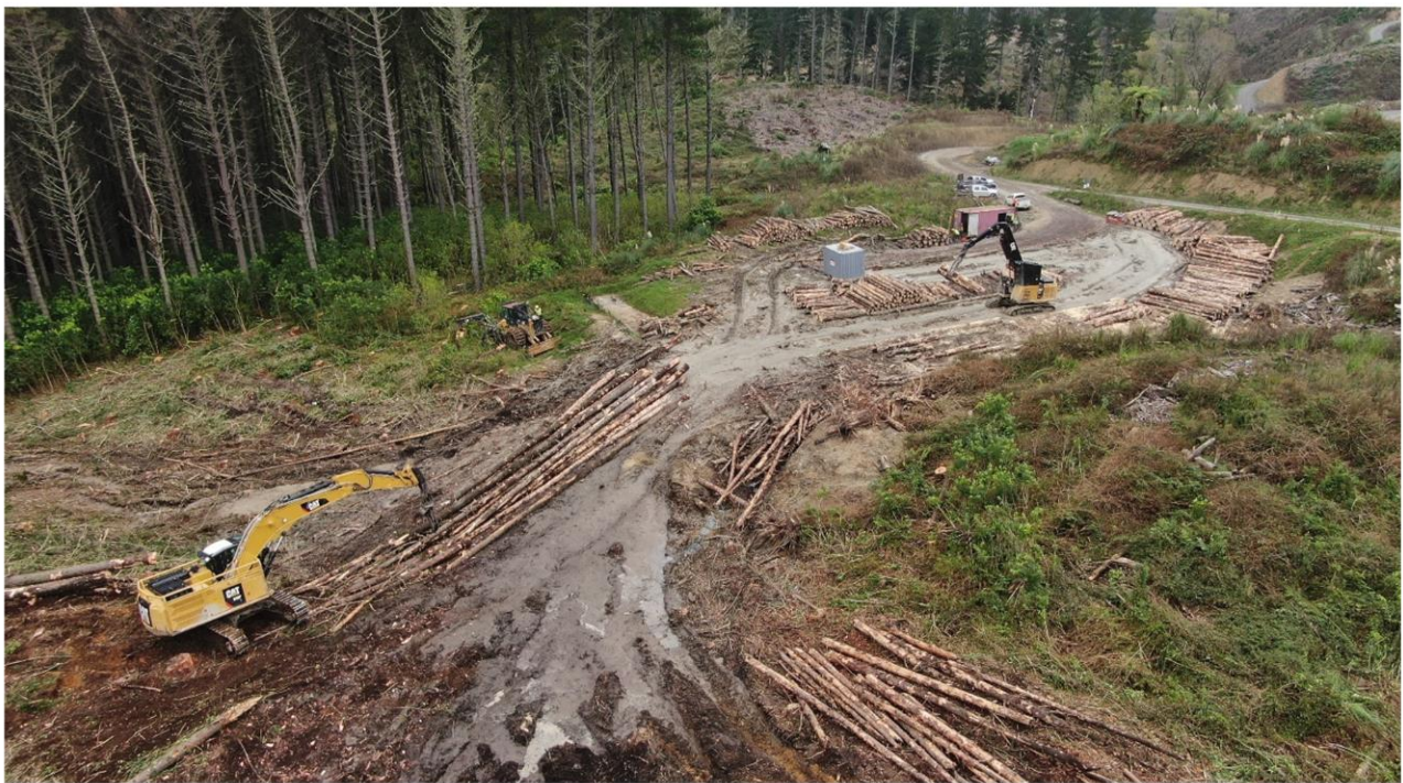
Setting 9, shovelling logs to landing to avoid environmental impact in rain.
