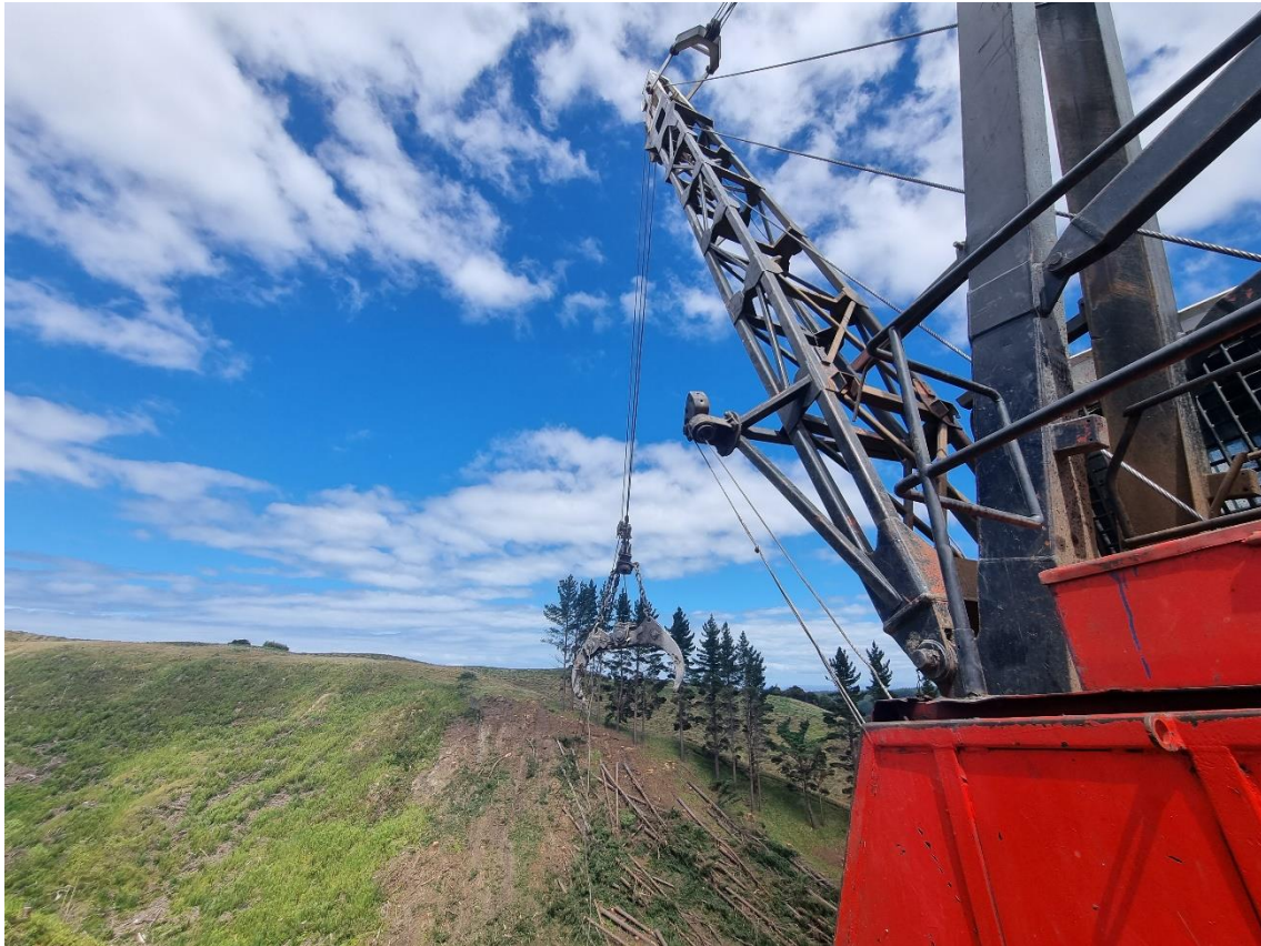
Photo 6: View from the swing yarder to the stems awaiting retrieval from the setting.
