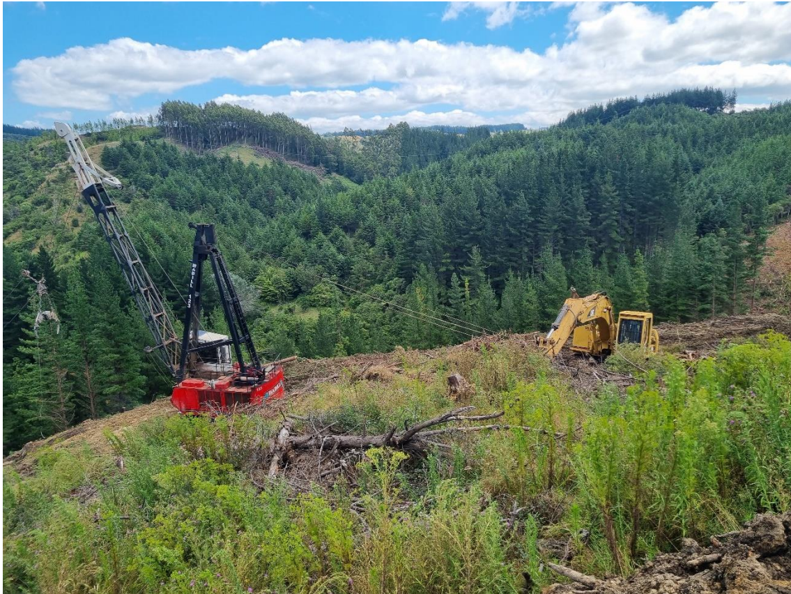
Photo 4: Swing yarder anchored by the excavator machine.
