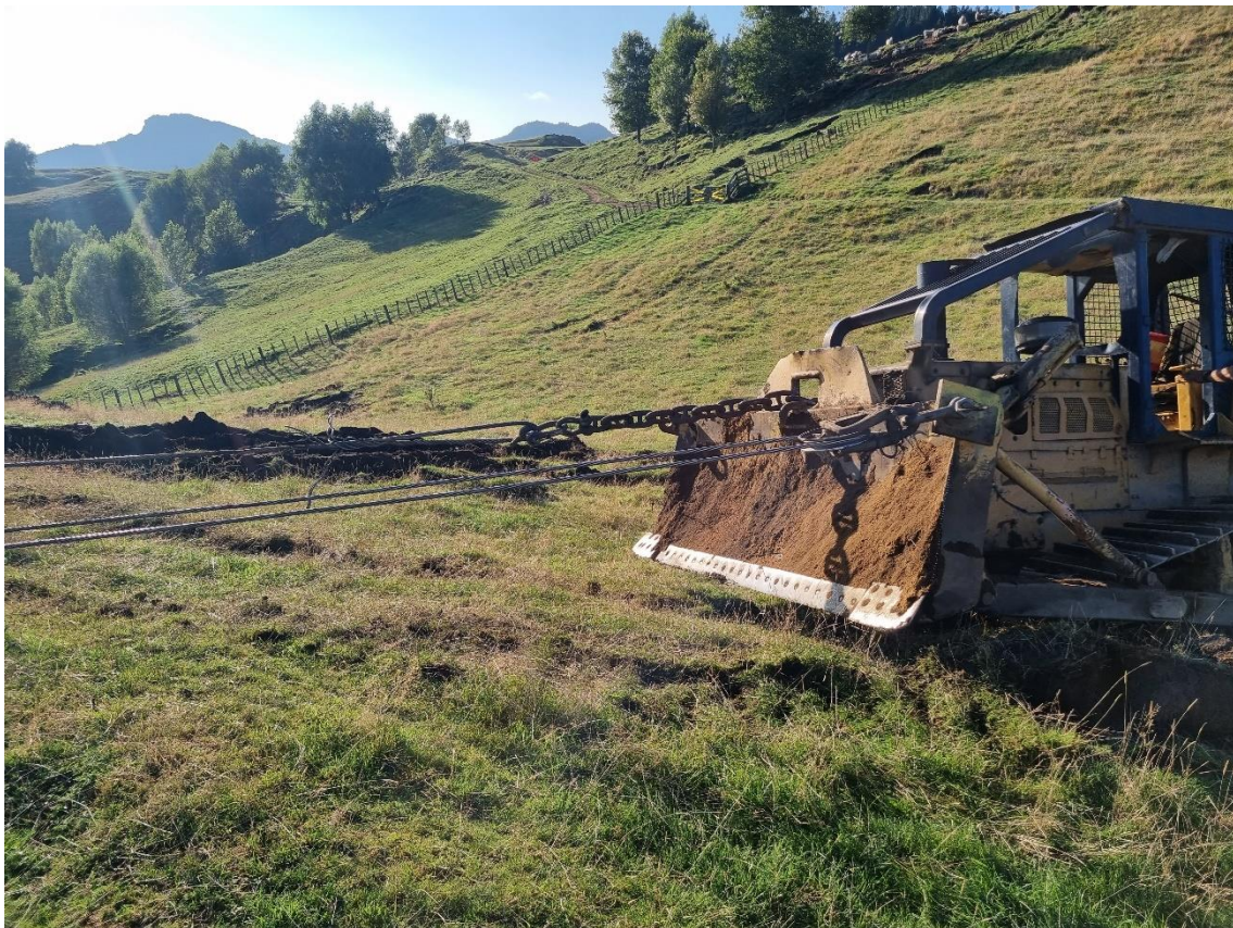
Photo 4: Looking at the blocks attached to the tail hold machine.
