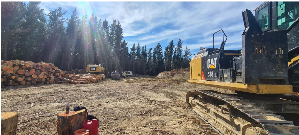
Photo 2: Machines being serviced, Landing 2.
