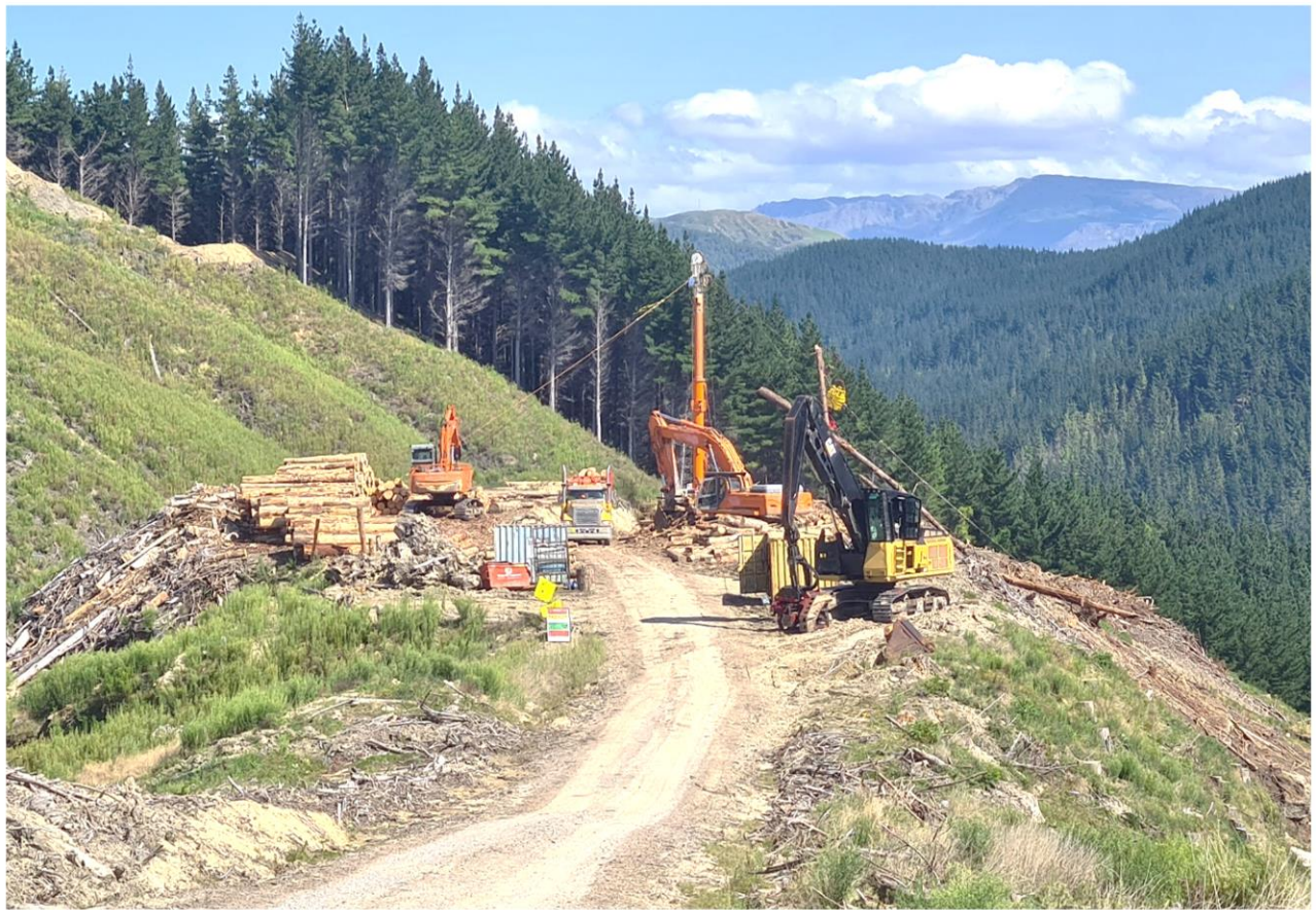
Loading out on Setting 4.
