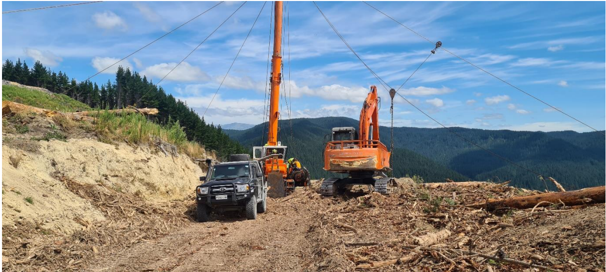
Photo 1: Swing yarder being repaired.
