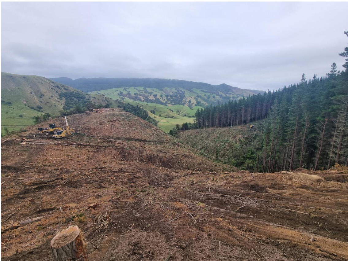
Photo 6: Haul setting area.
