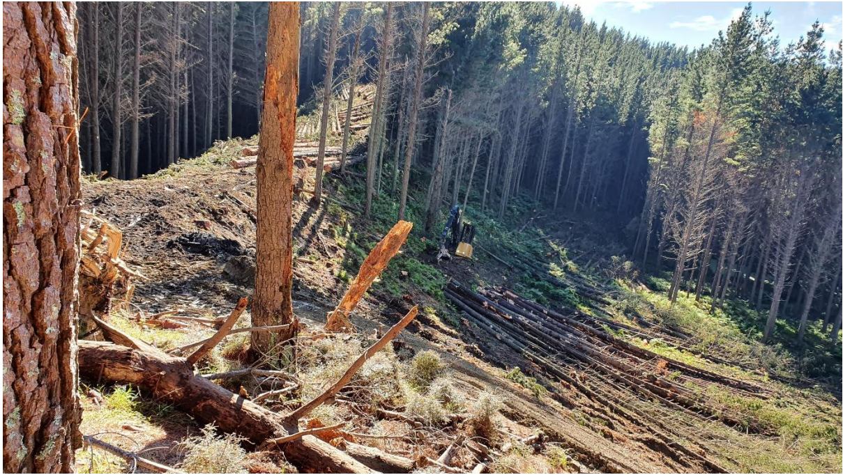
Photo 7: Roadlining area for Landing 23.
