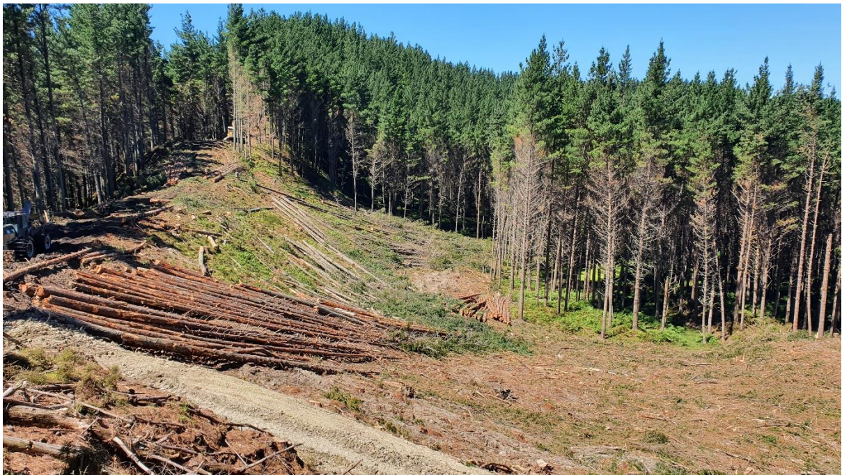
Photo 8: Setting 500 nearing completion of roadline for Landing 23 and Temporary Landing T2 construction.
