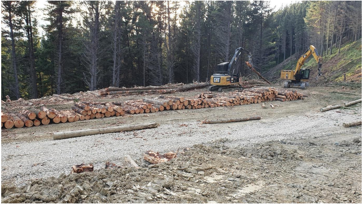
Photo 1: Roadlining Murry Road from Landing 22 to 23.
