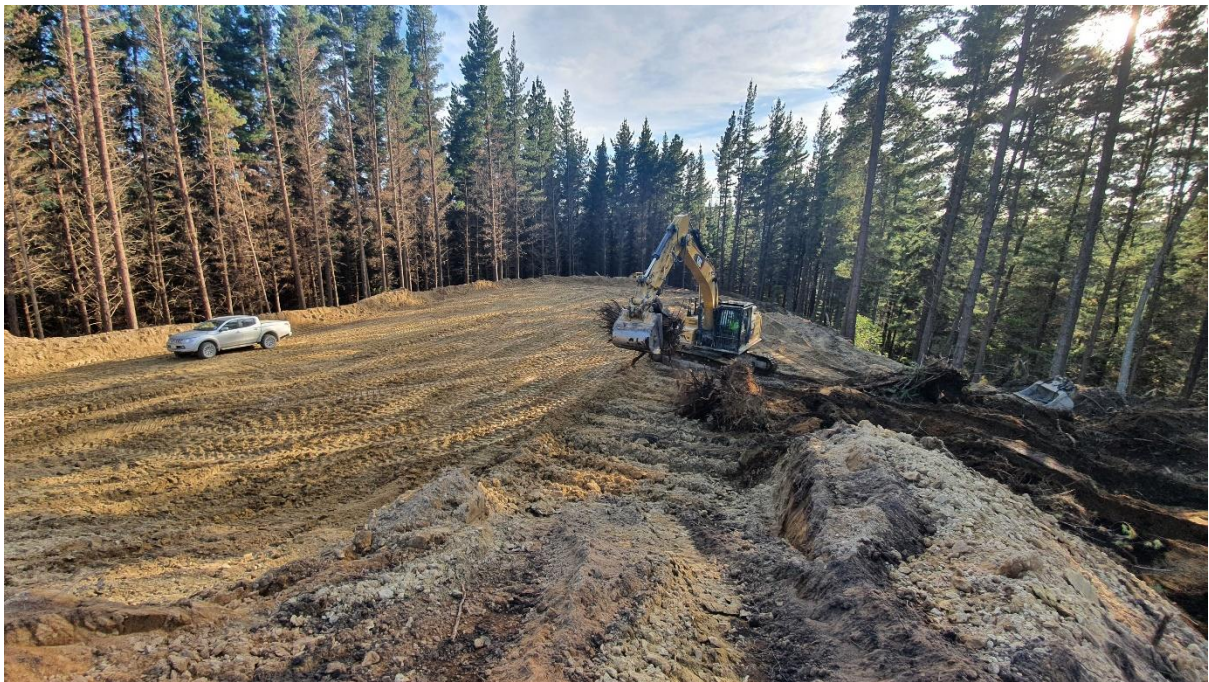
Photo 2: Earthworks crew de-stumping the two-stage track on the edge of Landing 18.
