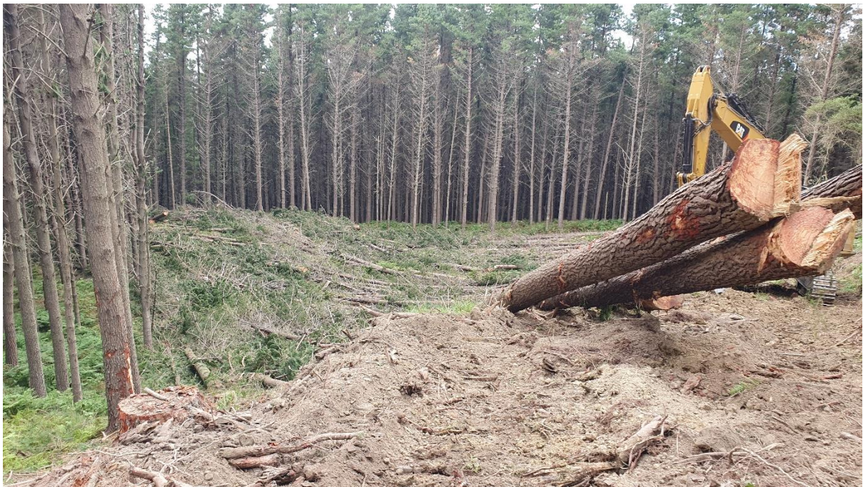
Photo 4: Roadline Setting 505, clearing the area for where Temporary Landing 2 will go.
