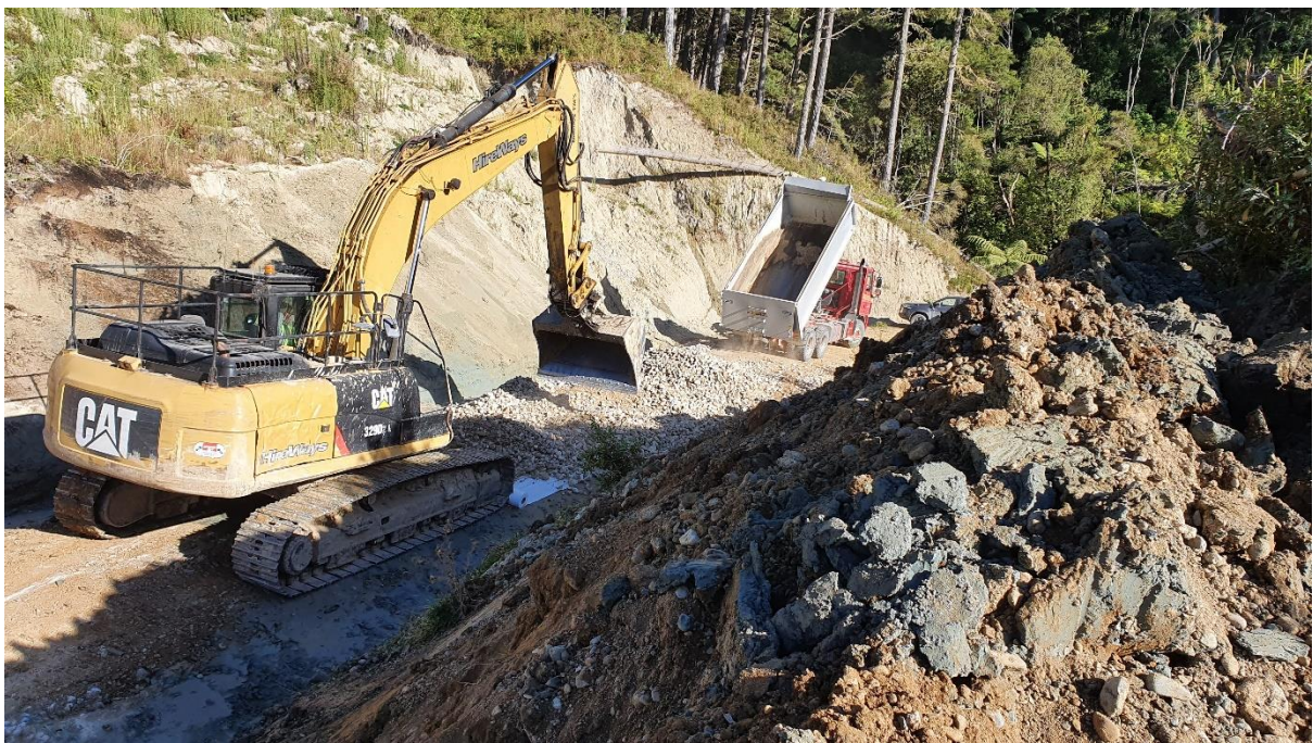
Photo 6: Roadline Setting 500, undertaking remedial works on a section of road that keeps failing.
